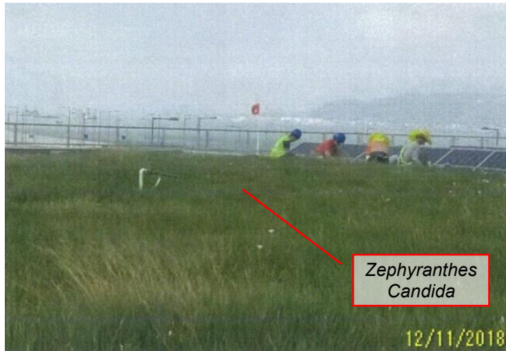
Building 023 roof greening (Photo 5 and Photo 6)
