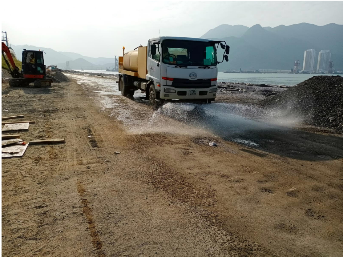
Photos of dust mitigation measures during the period of 4 – 6 Nov 2019
