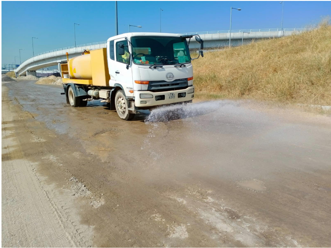
Photos of dust mitigation measures during the period of 21 – 23 Nov 2019
