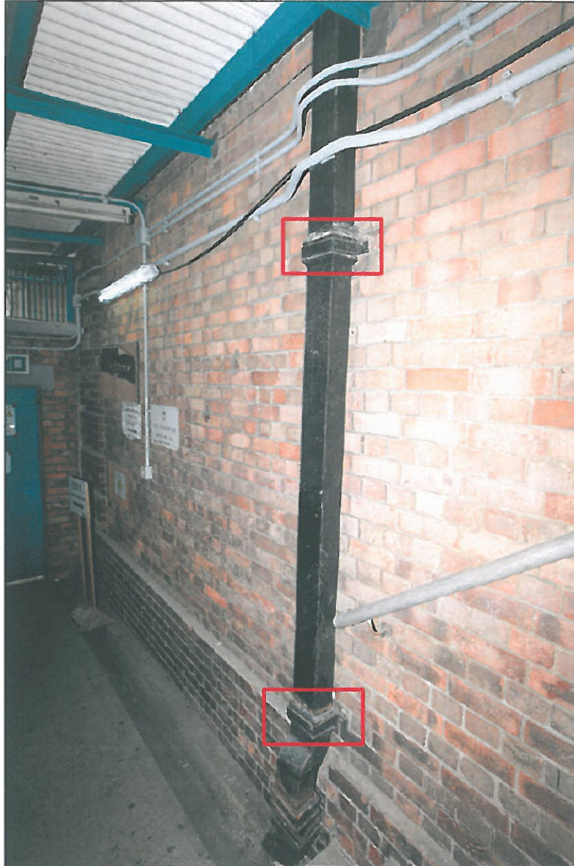
Photo 09-Ext-229 General view of the brick wall at the staircase to Block 09 (21-11-2011)
