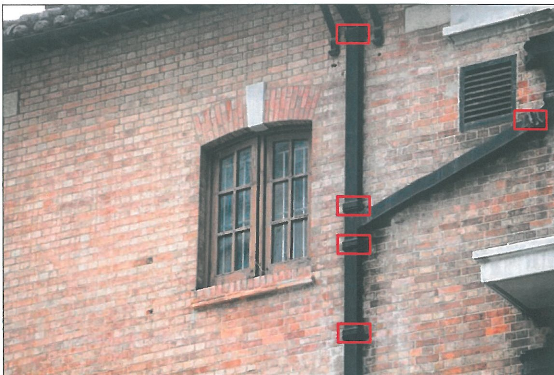
Photo 09-Ext-182 General view of the metal downpipes (17-8-2011)
