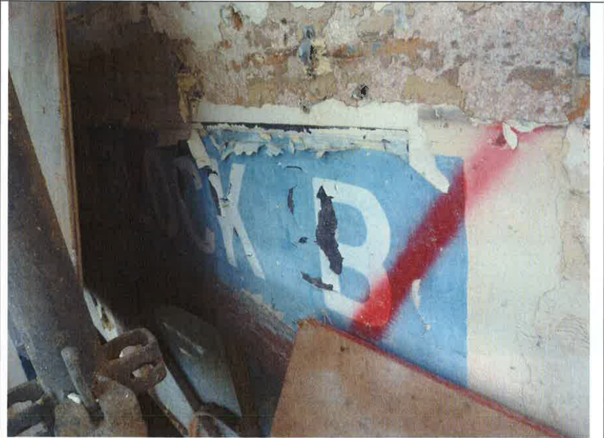
Block 04 South Elevation, photo was taken on 11/11/2014.
