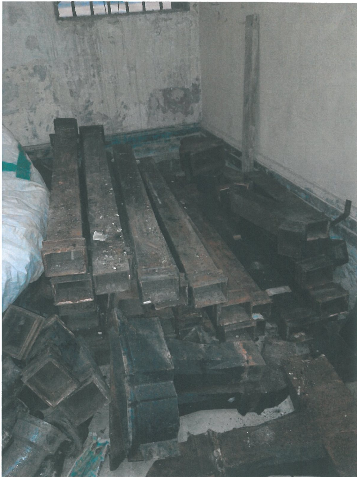
Above, photograph taken 30 September 2014 showing existing rain water goods from Block 9, only two holderbats were handed over, others assumed lost.
