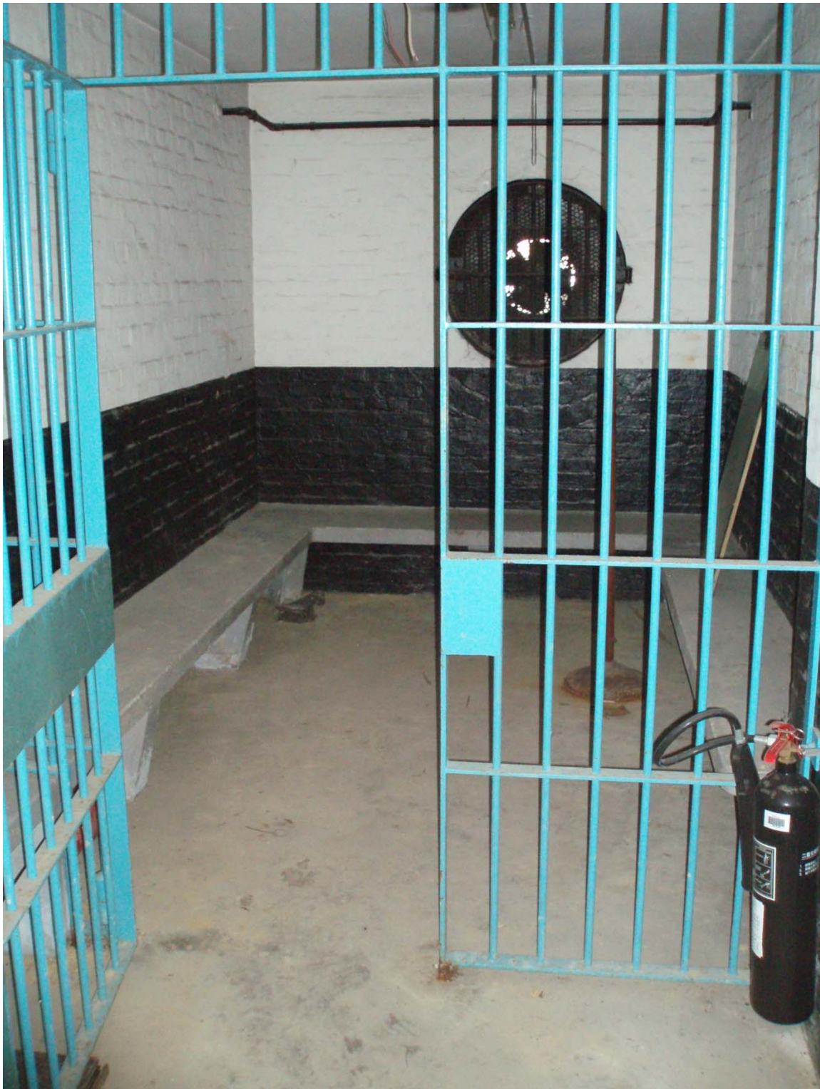
Above, photograph taken on 27 th July 2009, showing the overall look of the holding cell.
