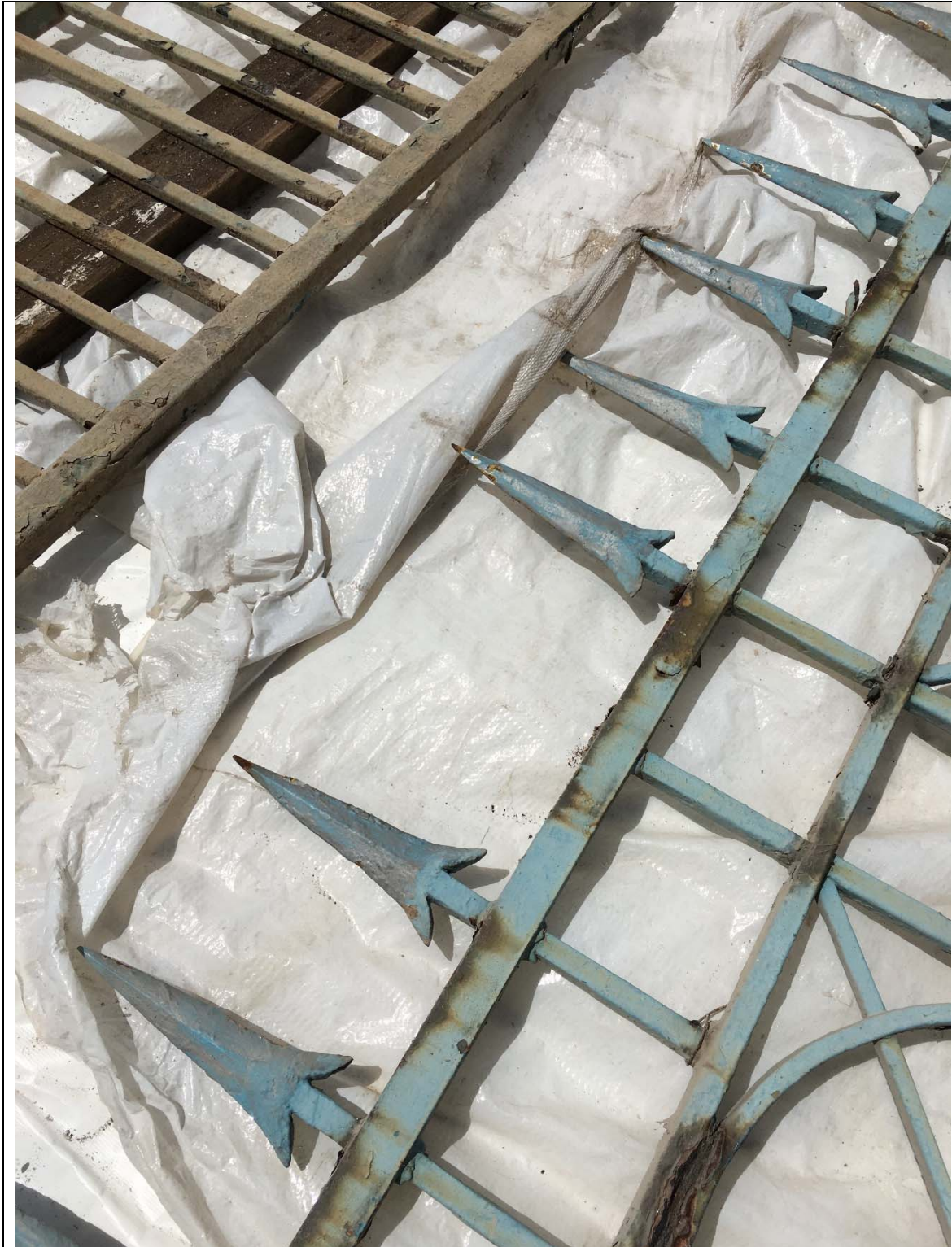
Above, photo taken on 21 st July 2016, showing one arrow on left hand side leaf was missing.
