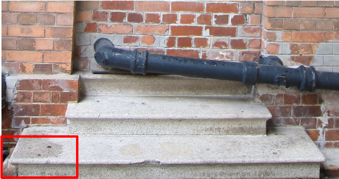
Above, photograph taken on 26 th April 2011, showing granite steps at 09/WG/04. The highlighted area was damaged during site works.
