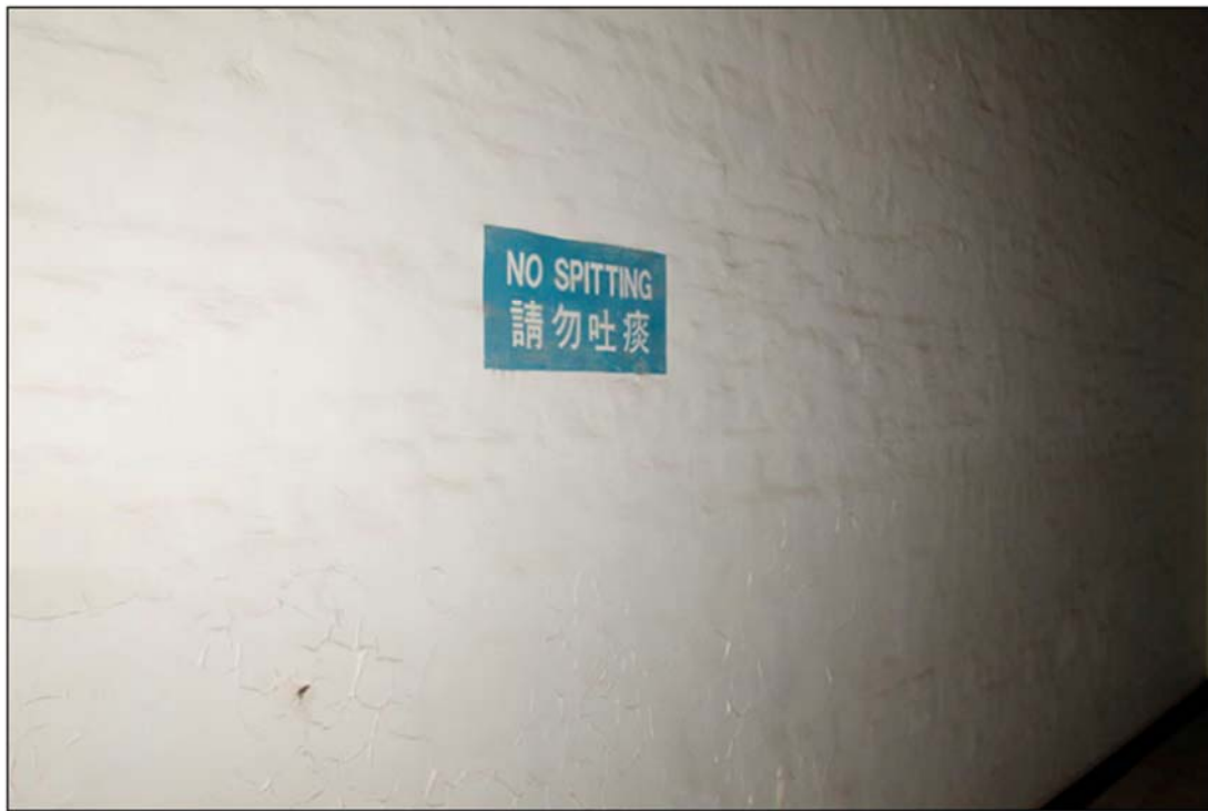
Photo 03-2F-230 General view of the wall (21-3-2012)
