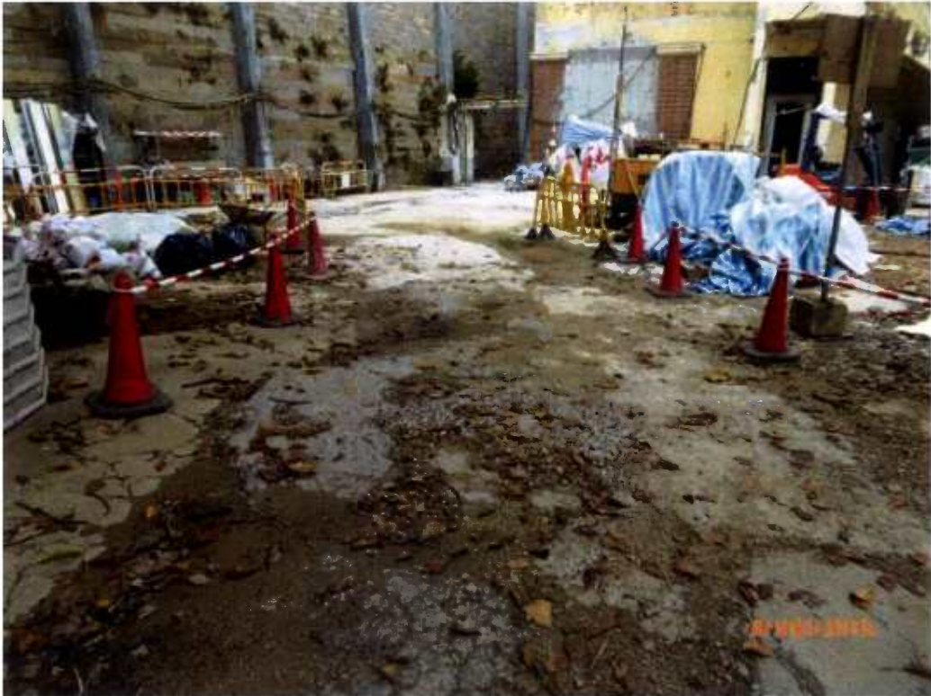
Fig. 10 Cleanliness of the site near Tree-6 is acceptable.
