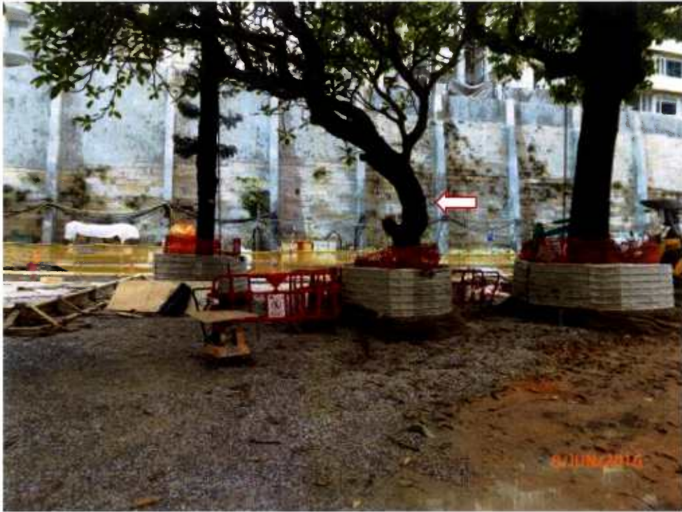
Fig. 8 Construction works are in progress near the tree.
