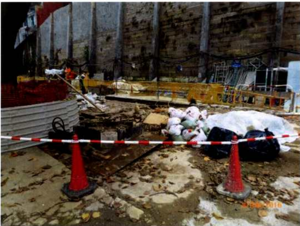
Fig. 11 Construction works are in progress near the tree.
