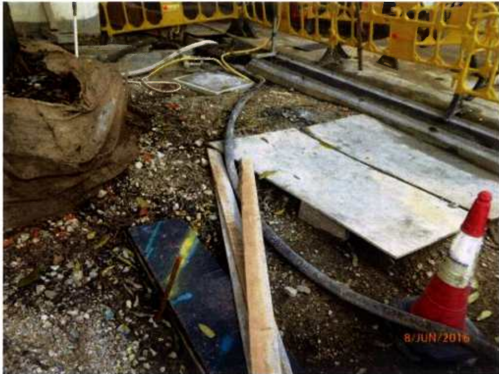
Fig. 10 Construction works are in progress near Tree-5.
