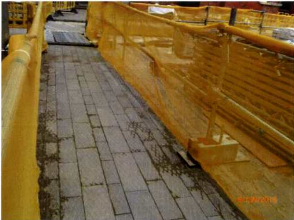
Fig. 11 The access near Tree-5 appears clean and tidy.
