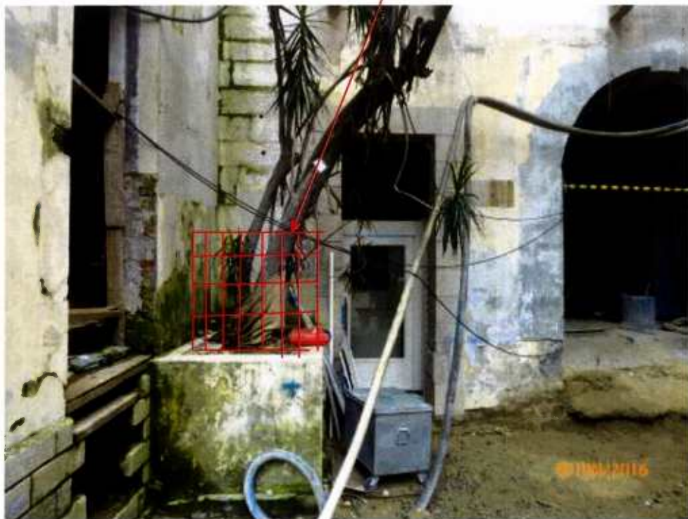
Fig. 3 Recommend to set up a small cordon zone to protect the tree.
