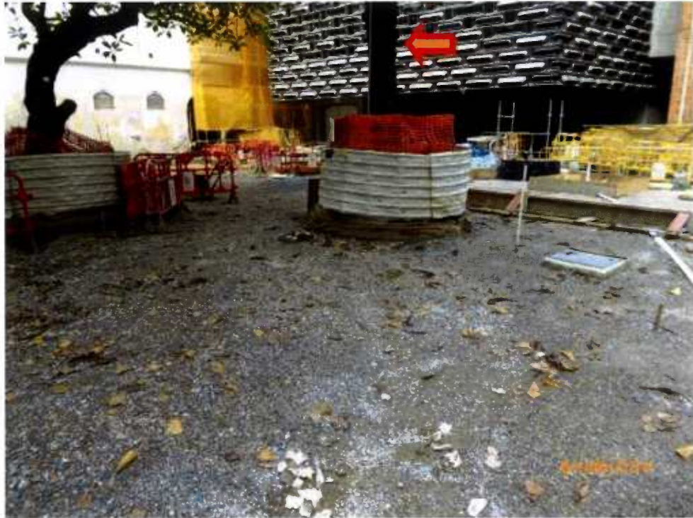
Fig. 10 Construction works are in progress near Tree-9.
