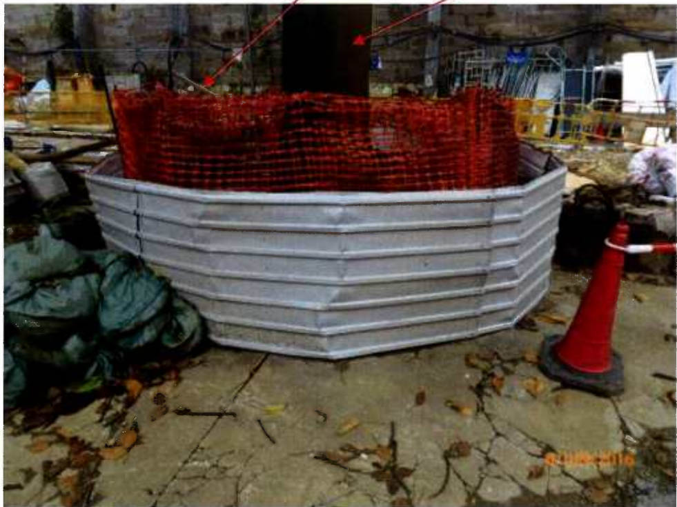
Fig. 3 Recommend to set up a cordon zone (similar to Tree-6 ) to protect the tree.
