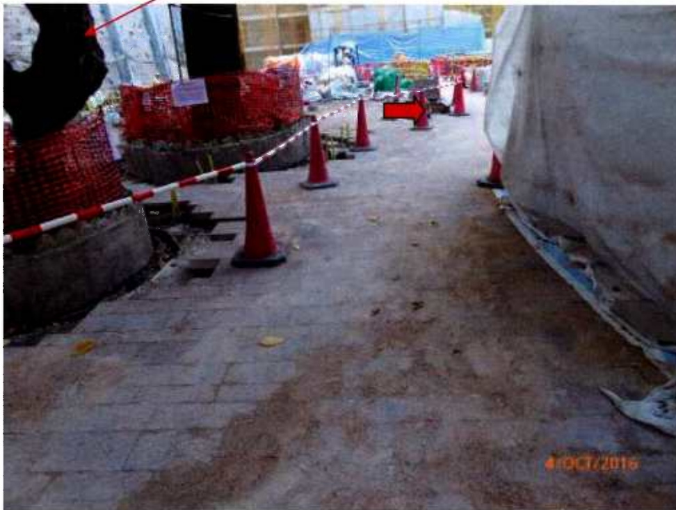
Fig. 11 Access near Tree-8 is clean and tidy.
