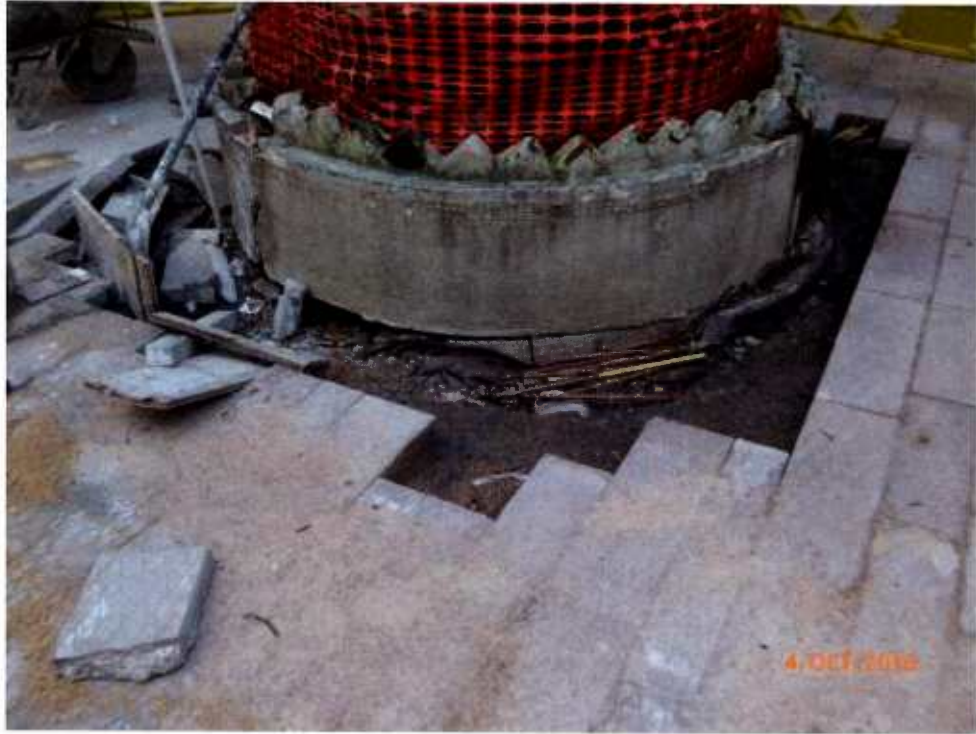
Fig. 10 Renovation works are in progress near the planter.
