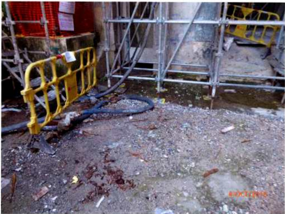
Fig. 11 Cleanliness of the site near the tree is acceptable.
