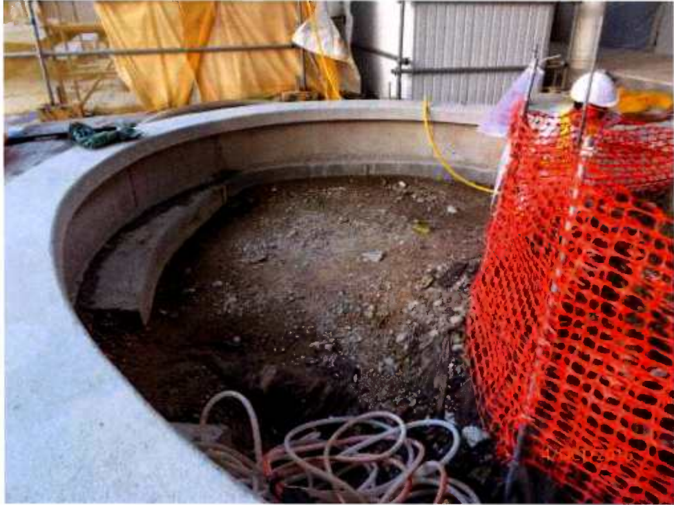
Fig. 10 The newly built planter is ready for backfilling of topsoil.
