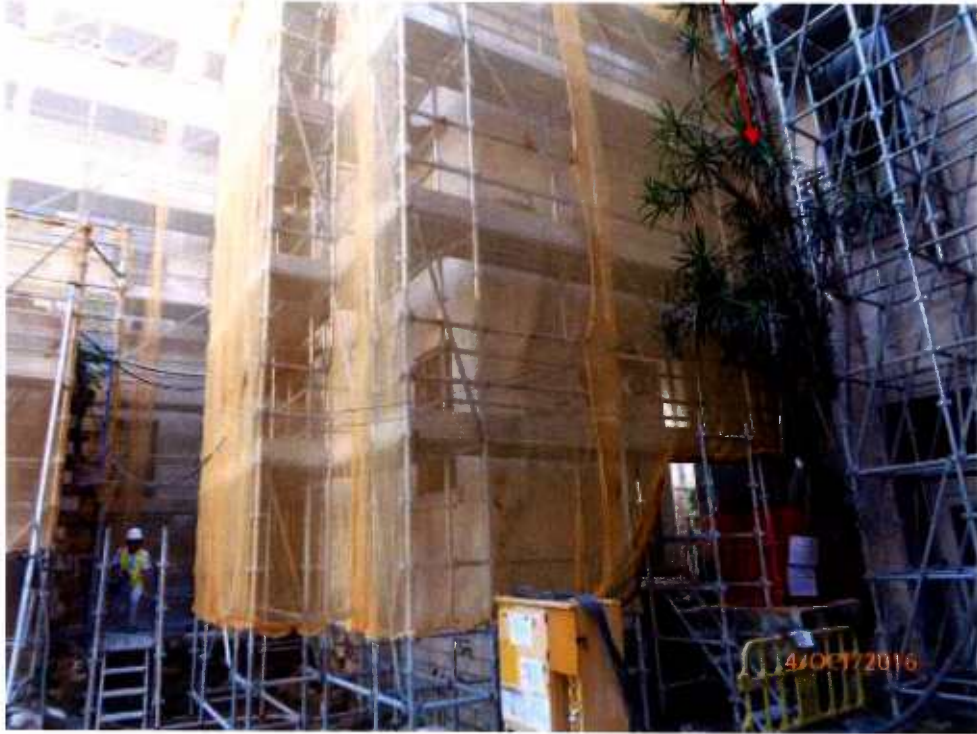
Fig. 10 Renovation works are in progress near Tree-11 .
