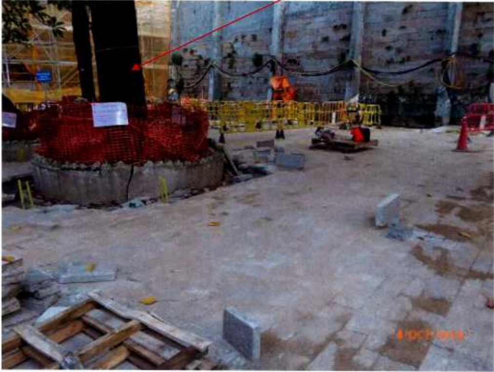
Fig. 10 Renovation works are in progress near Tree-7 .
