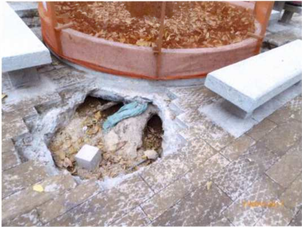
Fig. 10 Four pits were recently excavated close to the planter.
