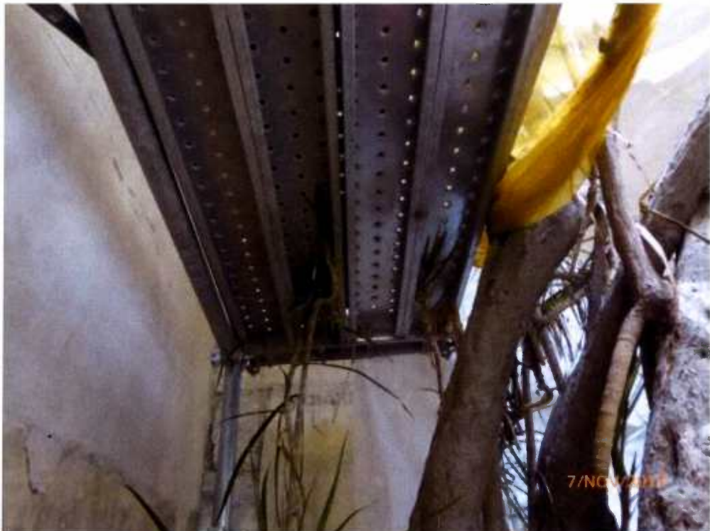
Fig. 7 The metallic platform is continuously set up close to the tree.
