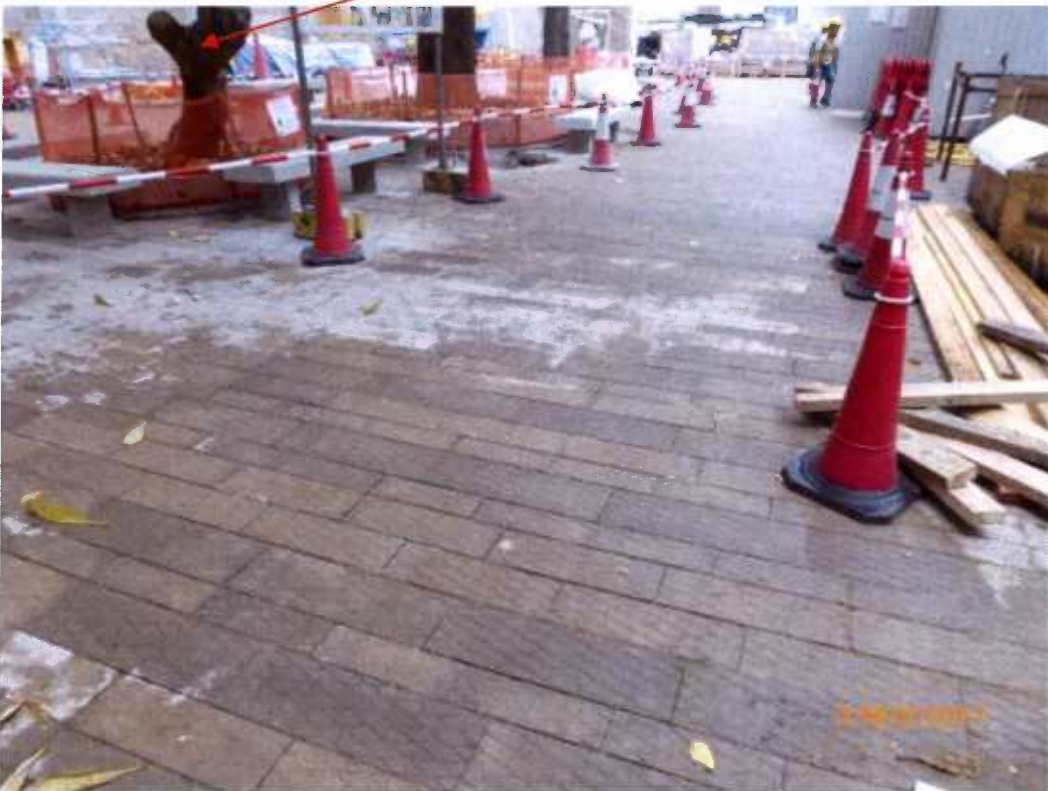
Fig. 11 The access near Tree-8 also is clean and tidy.
