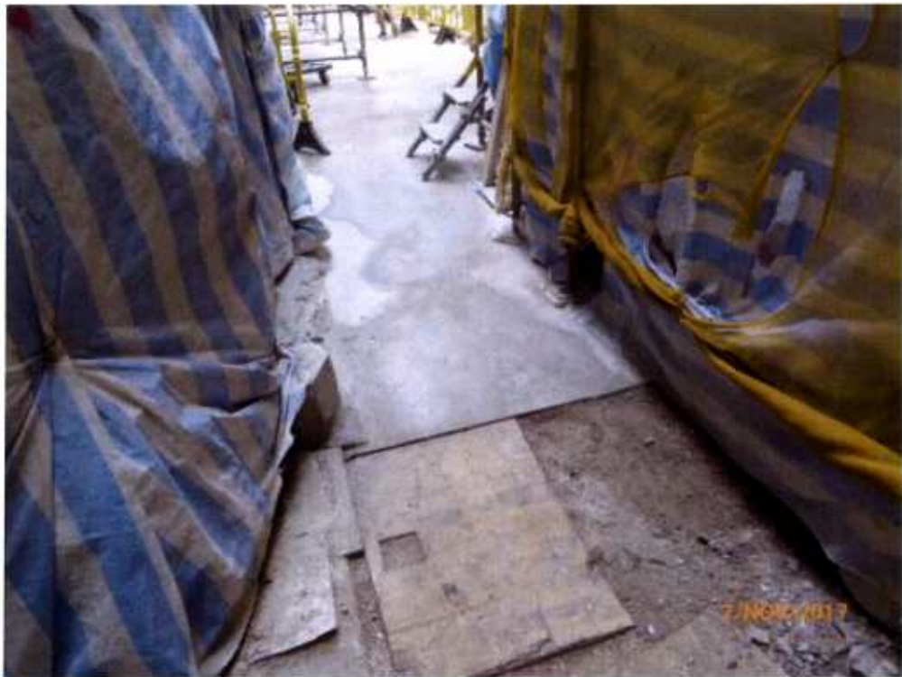
Fig. 11 Cleanliness of the nearby access is acceptable.
