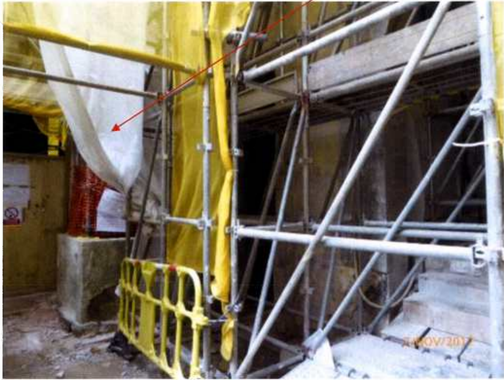
Fig. 10 Renovation works are in progress near Tree 11
