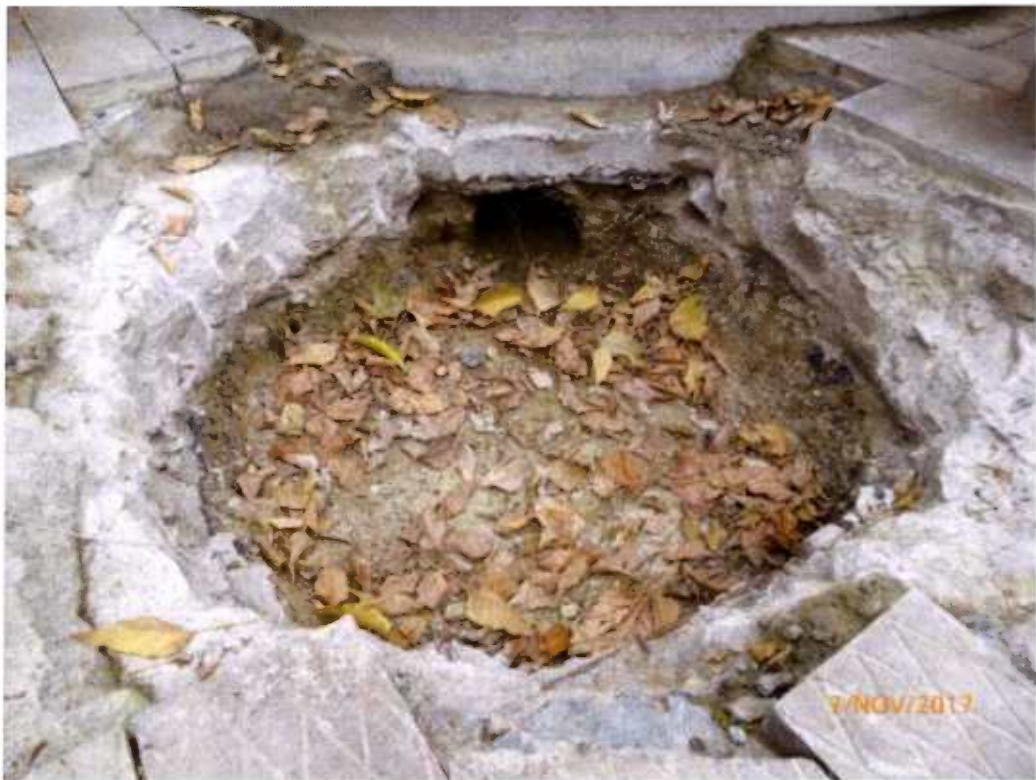
Fig. 11 Four large pits have been excavated close to the planter.
