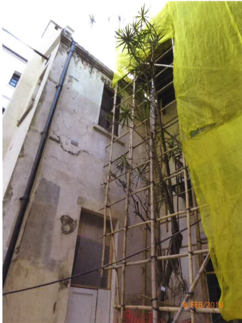
Fig. 12 Overall view of Tree-11 during inspection on 8 th February 2018.
