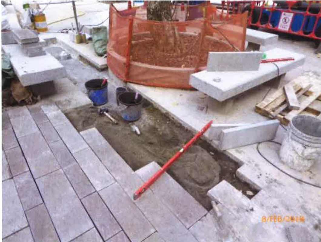
Fig. 10 Renovation works are in progress near Tree-8.
