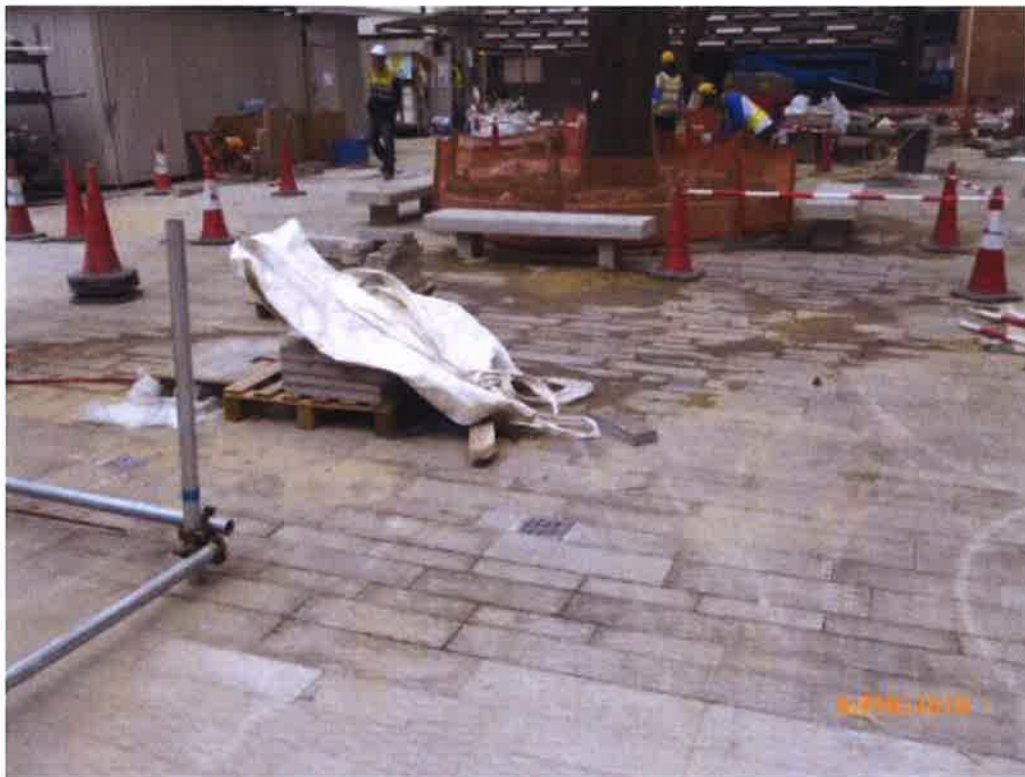
Fig. 11 Renovation works are in progress near the tree.
