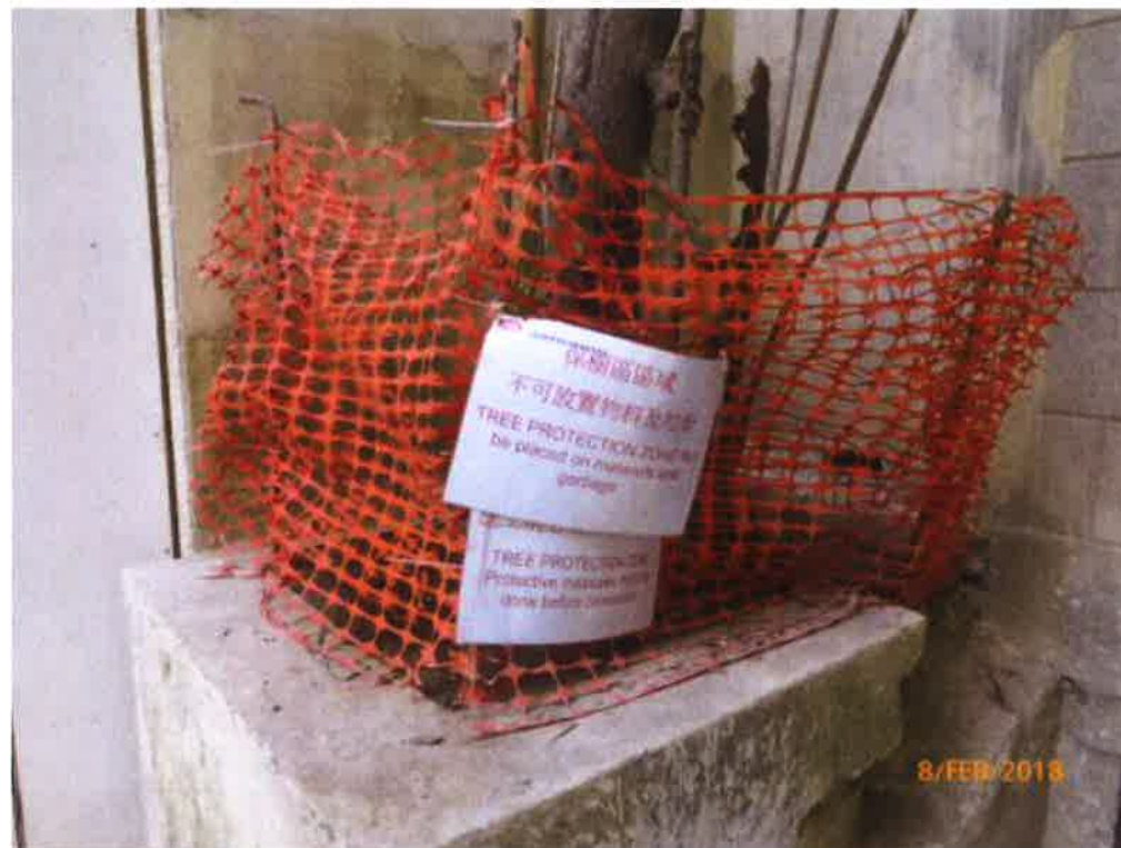
Fig. 9 The tree protection zone is in order.
