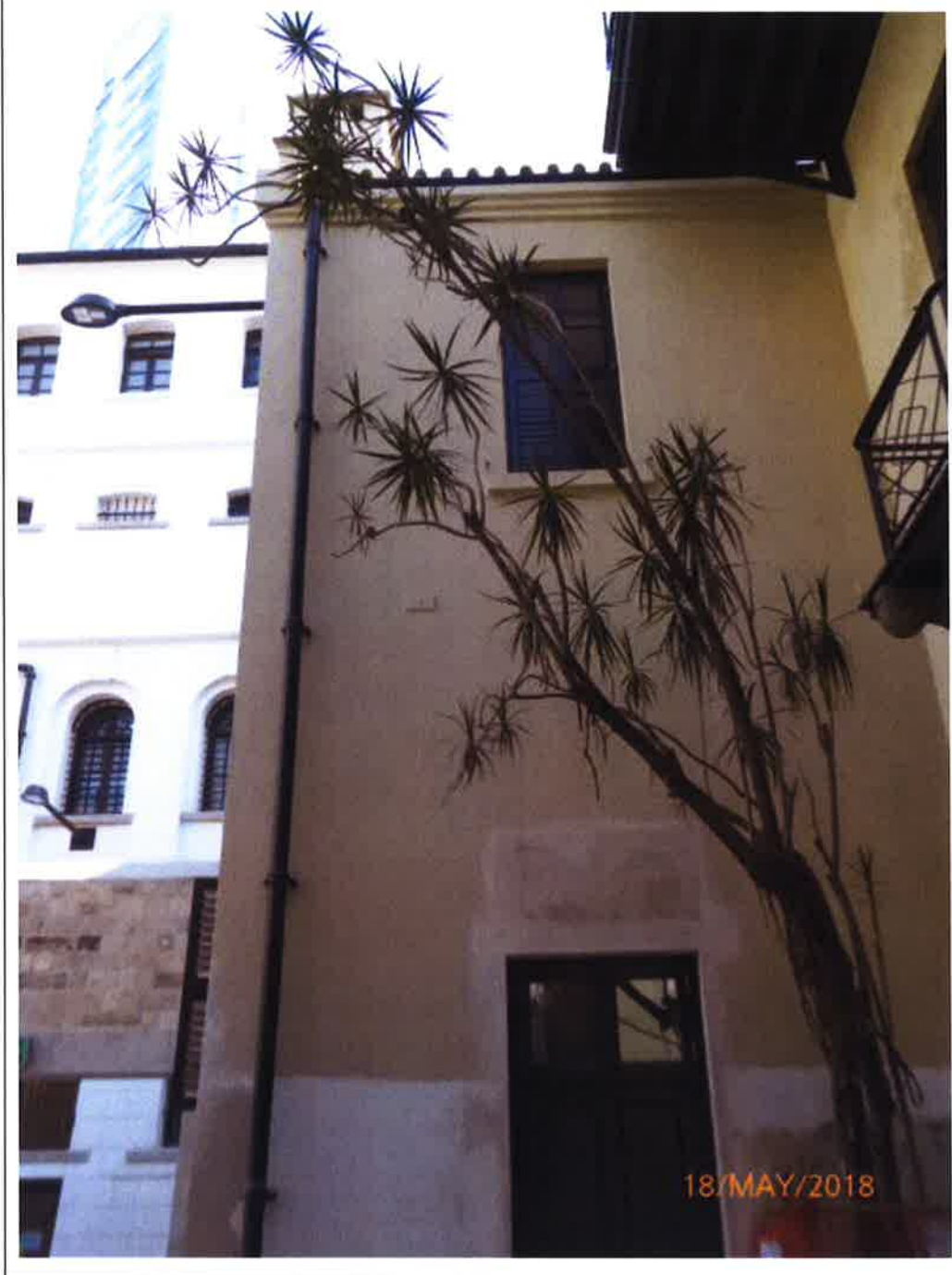
Fig. 12 Overall view of Tree-11 during inspection on 18 th May 2018.
