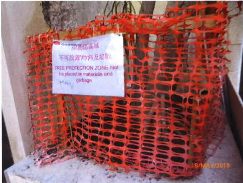
Fig. 10 The tree protection zone is in order.
