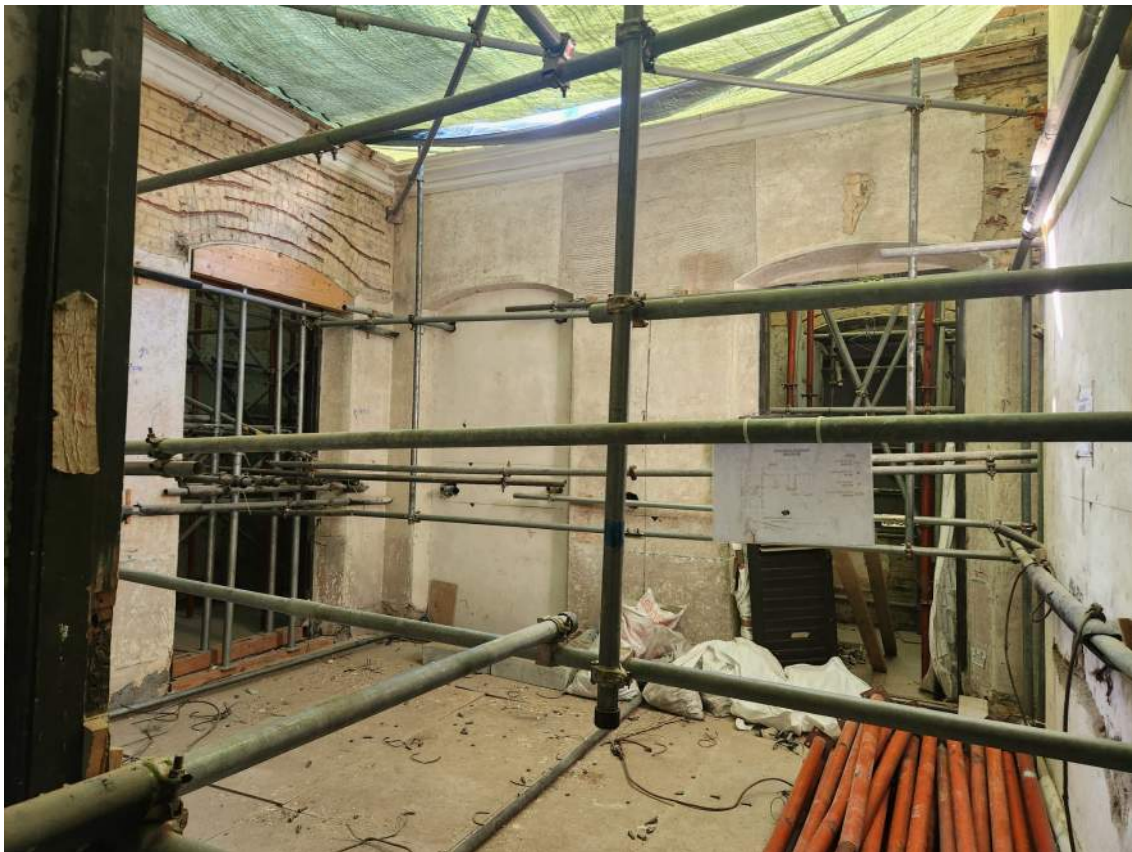
Figure 3 - Second main room with all vertical props removed on site
