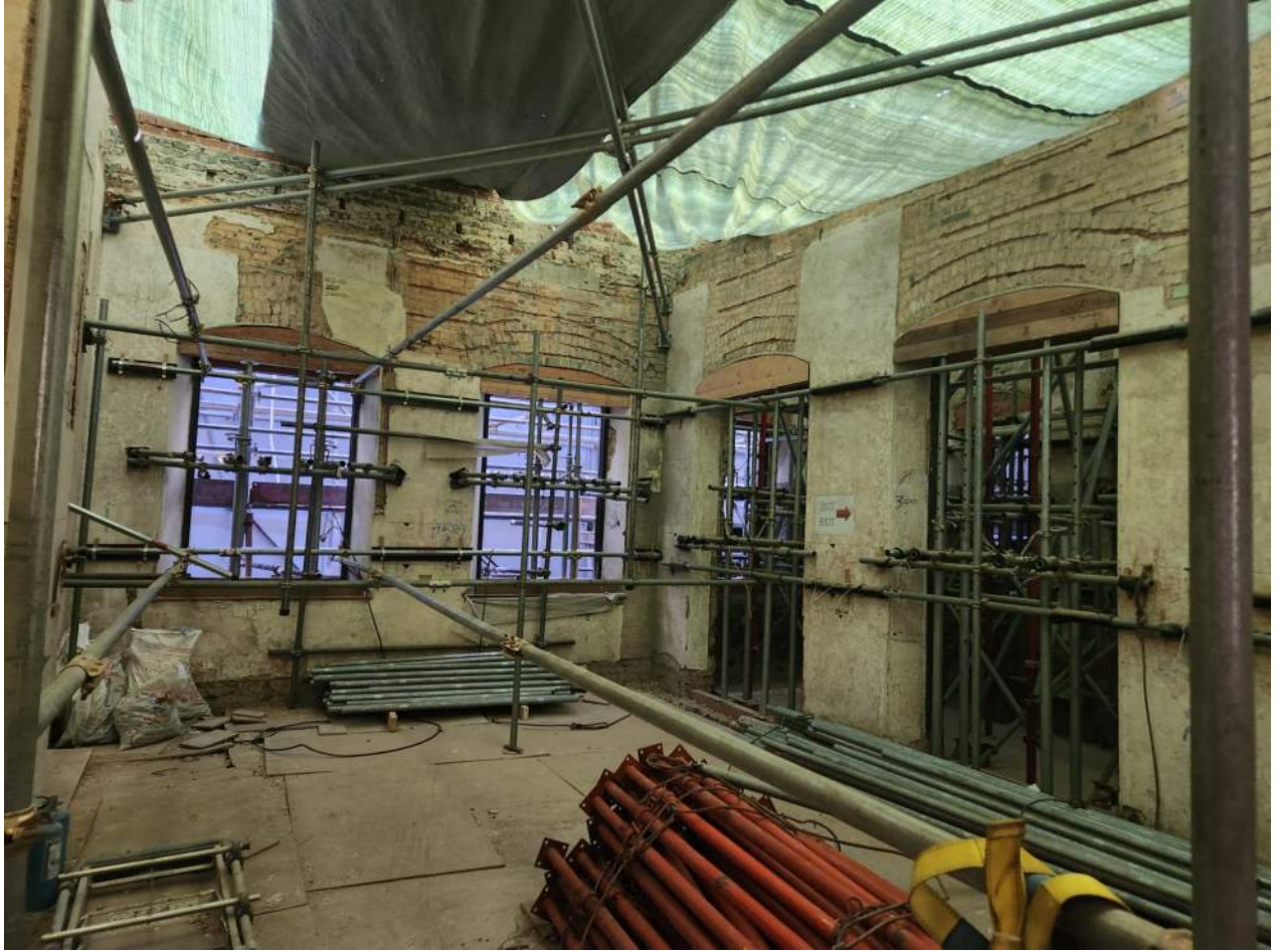
Figure 2 – Main room with all the vertical props removed on site
