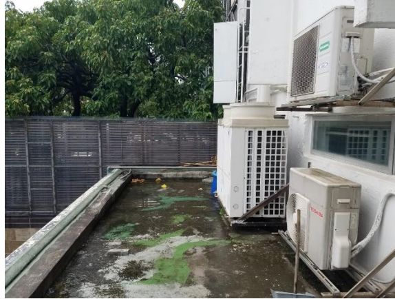
Construction Dust Monitoring Location
