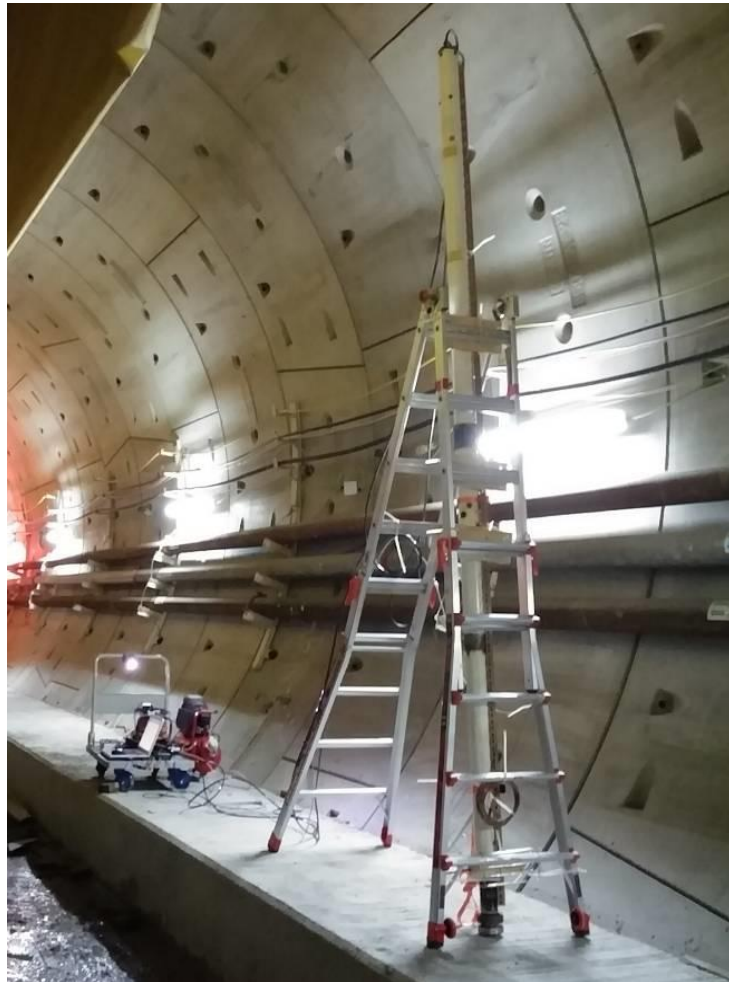
Hammer Impact Test in the Tunnel
