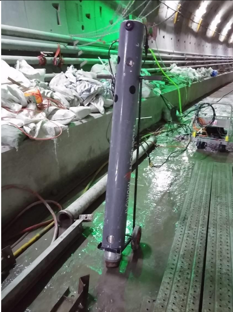
Hammer Impact Test in the Tunnel
