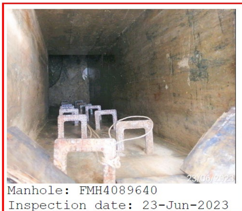
Photo 2 – Condition of Blocked Manhole after removal of rubbish and debris
