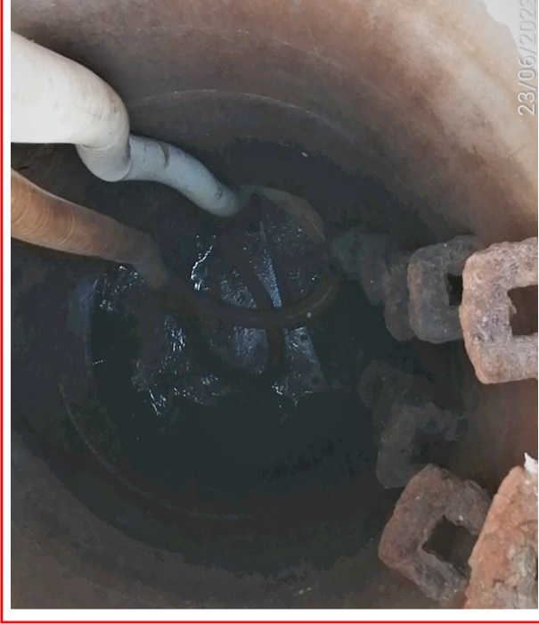
Manhole: FMH4038041 Inspection date: 23-Jun-2023 Remark: DN825 diversion in progress
