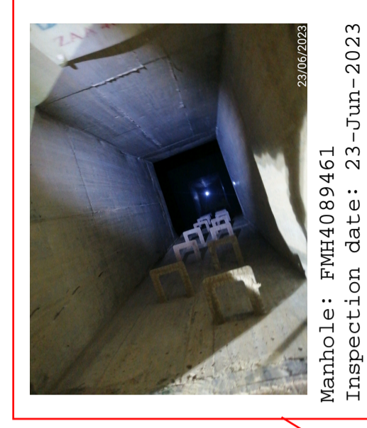
Manhole: FM8 Inspection date: 23-Jun-2023
