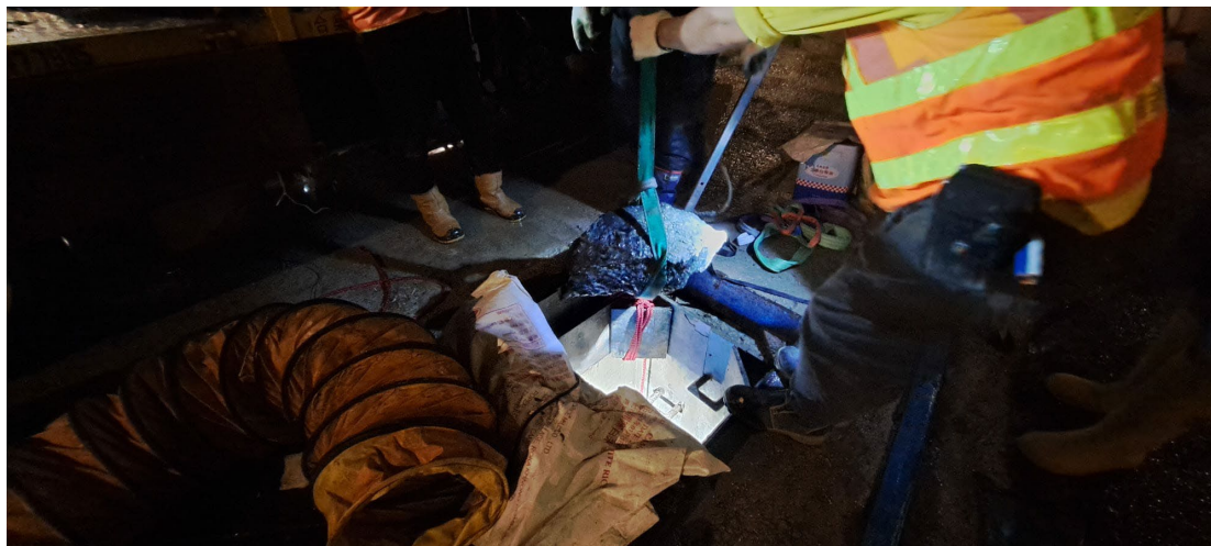
Photo 2 – DSD continued coring between existing sewage manholes at slow lane (photo date: 17^18/6/2023 and photo provided by DSD)
