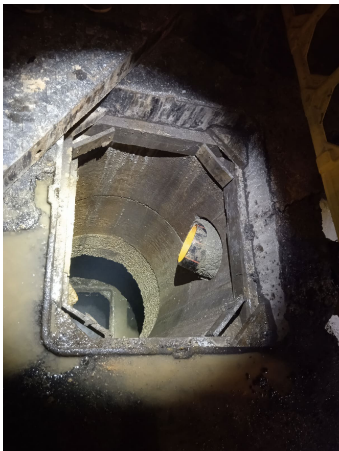
Photo 3 – by pass pipe constructed by CCZJV at FMH4038025
