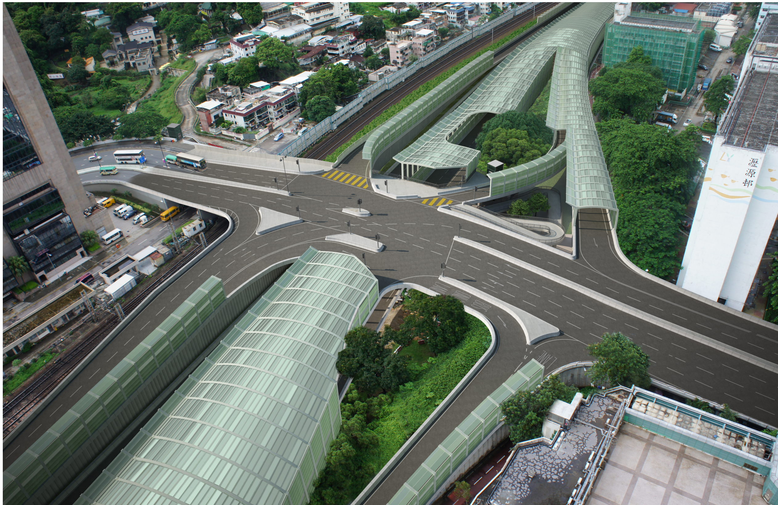
View 1: Proposed Diamond Shaped Interchange at Junction of Tai Po Road (TPR) / Sha Tin Rural Committee (STRC Road)
