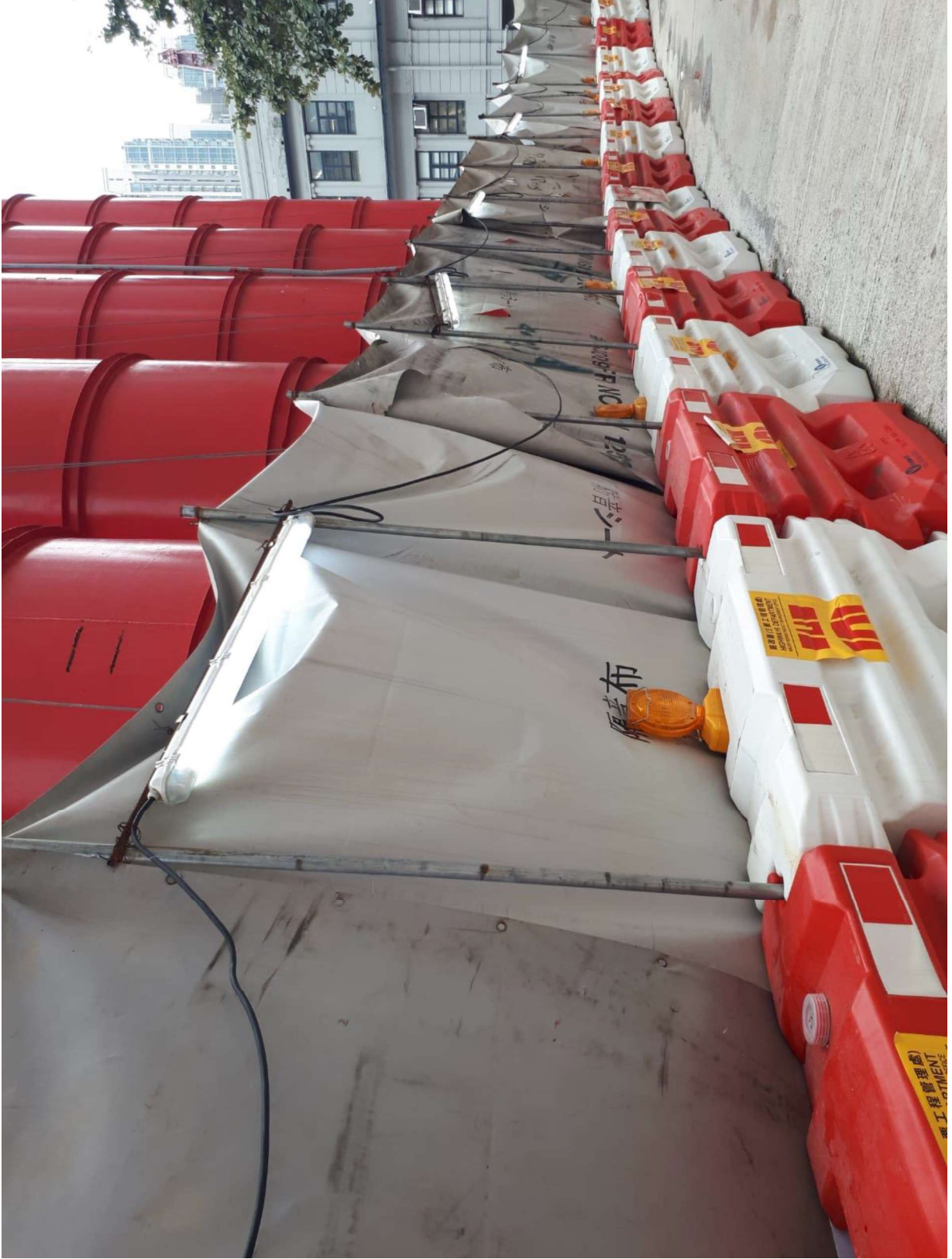
Remark 2: Noise barrier at Zone D3
