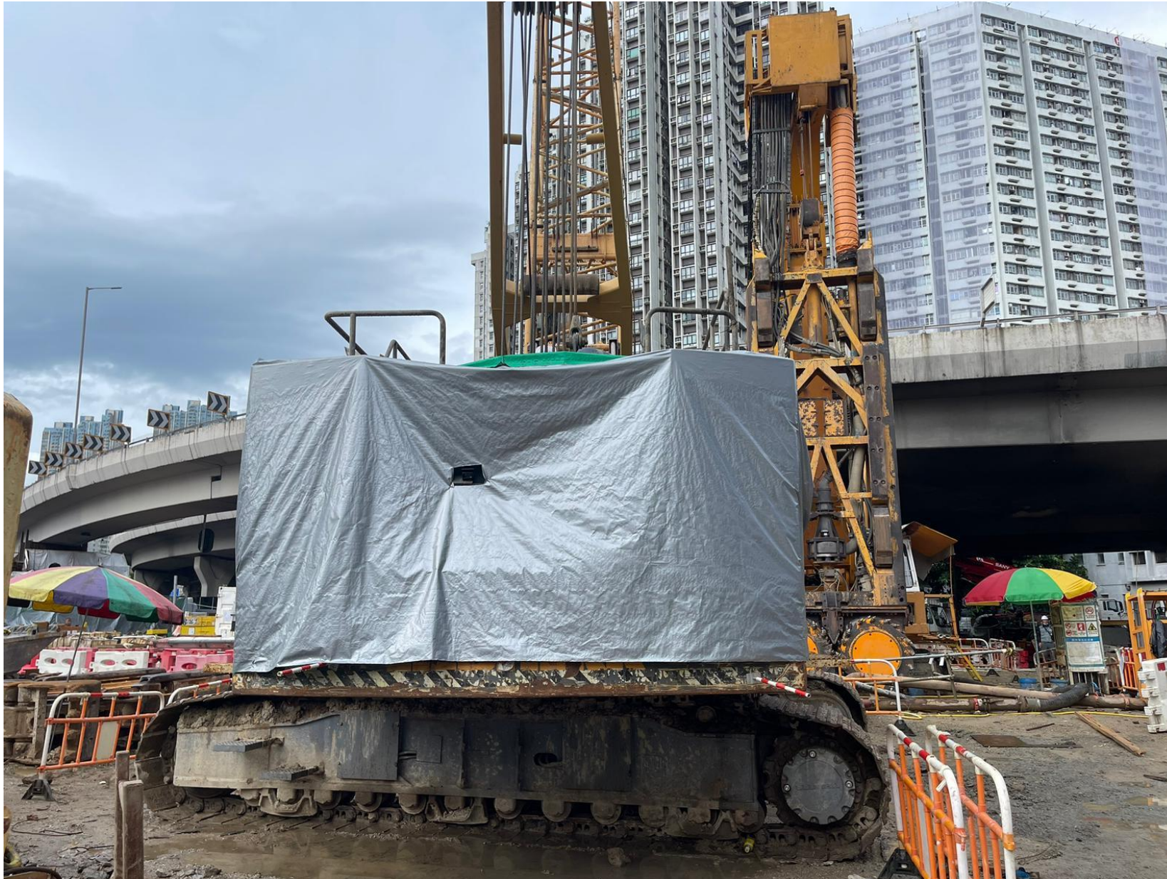
Remark 3: Additional noise canvas at the engineering part of the mobile crane
