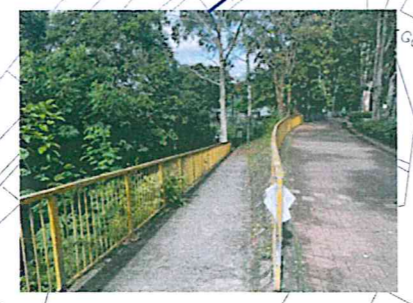
Water barriers will be provided during the roadworks construction under TTA submission.
