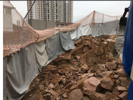
Photo 3 Repaired noise barrier near Slope H
