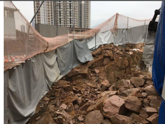
Photo 3 Repaired noise barrier near Slope H
