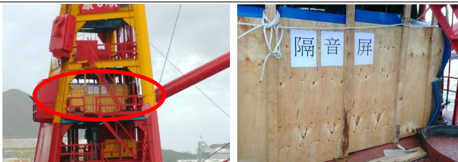
Figure 1 Erection of noise barrier on the barge
