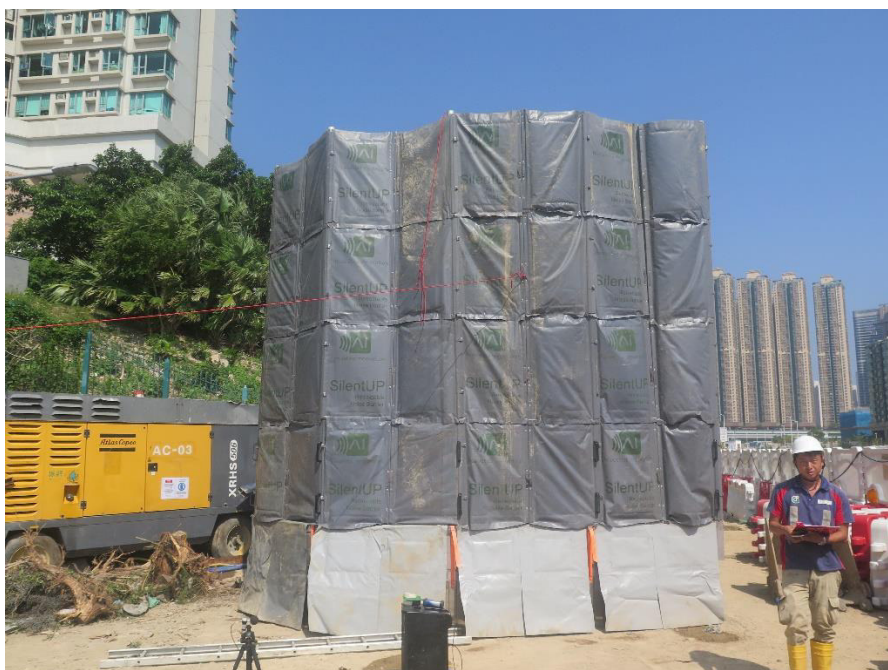
Photo 1. Noise Barrier (front view)
