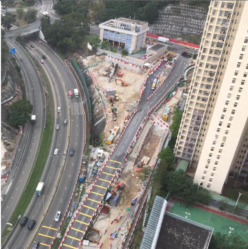
Photo 2 PMEs distribution at Portion IVC
