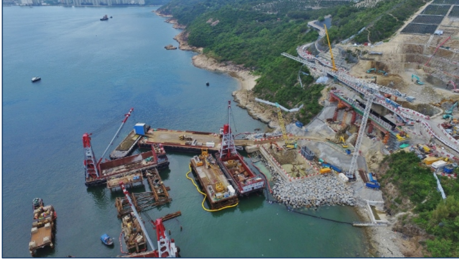
TKO - Lam Tin Tunnel - Main tunnel and associated works using DSP silt curtain
