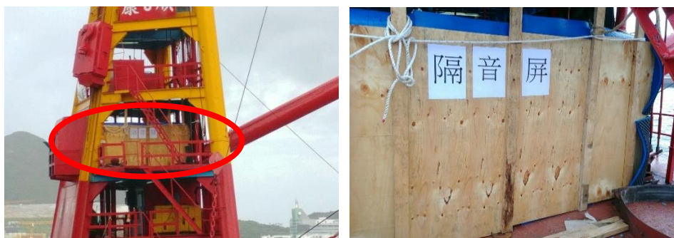
Figure 1 Erection of noise barrier on the barge
