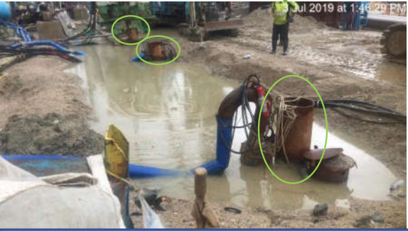
600mm dia. Soak Away Pit -14mPD (Portion 9)
