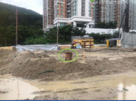
600mm dia. Soak Away Pit -14mPD (Portion 9)
