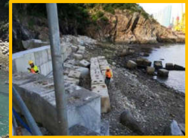
Extension of Sed tanks
