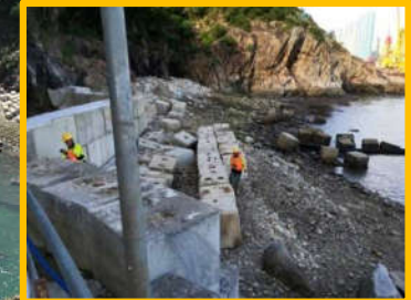
Extension of Sed tanks
