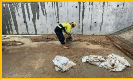
Site Clearance & provide cover to exposed excavation area
