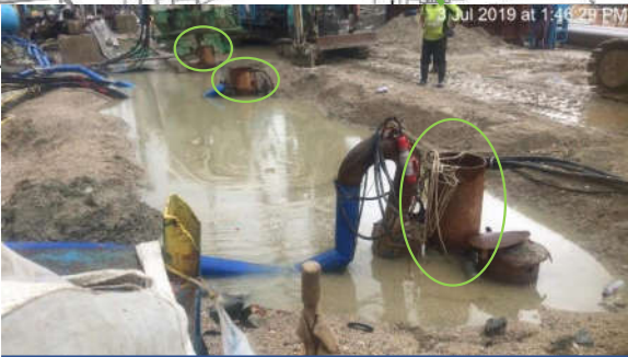
600mm dia. Soak Away Pit -14mPD (Portion 9)
