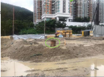
600mm dia. Soak Away Pit -14mPD (Portion 9)
