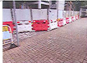
Sandbag is placed along the water barrier boundary to avoid the surface runoff.
