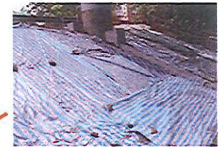
Exposed slope is covered by taupaulin
