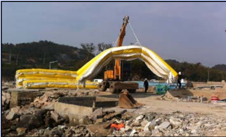
Handling of the silt curtain
