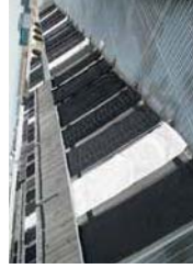
Outdoor Exposure Test
