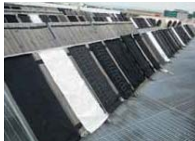
Outdoor Exposure Test
