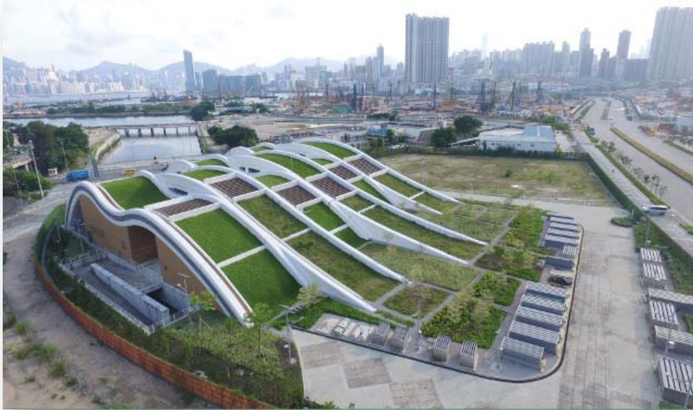
Kai Tak Development - Reconstruction and Upgrading of Kai Tak Nullah
