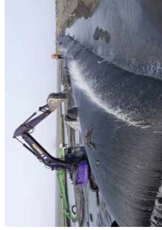
ACEGrid® Geotextile Mattresses for Separation and Erosion Control
