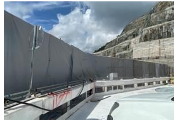
Photo 4 (Provided by Contractor)
