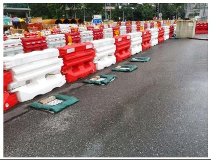
Gully were protected and covered by geotextile.
