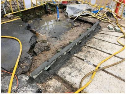
Height difference between the road and site area to form a natural flow. Sump pit was provided for wastewater collection.
