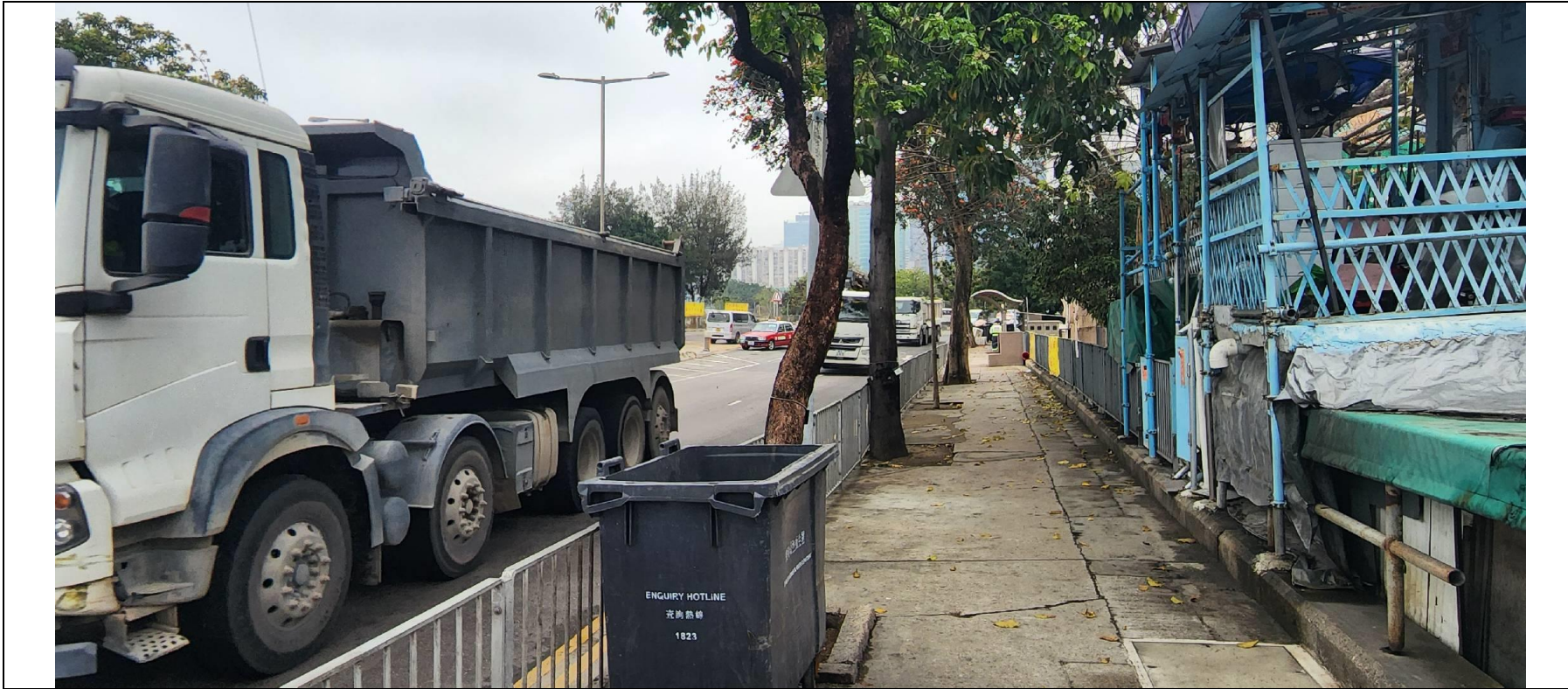
Photo 3 – Road condition along Cha Kwo Ling Road next to station AM4(B) (Taken on 18 Mar 2023)
