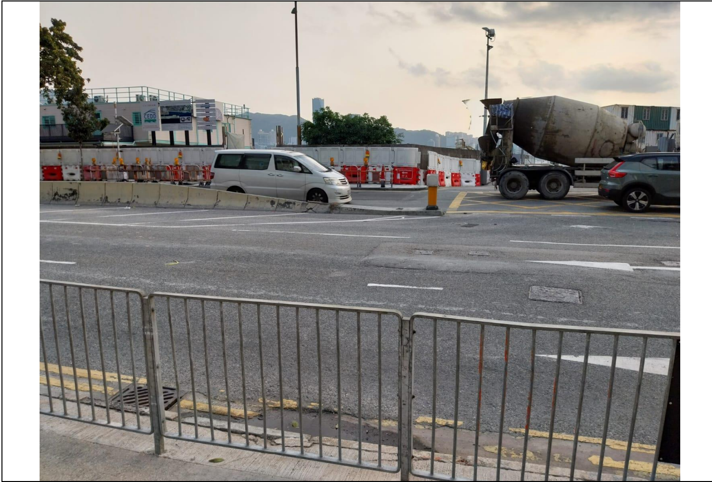
Photo 4 – Road condition along Cha Kwo Ling Road next to station AM4(B) (Taken on 02 Mar 2023)
