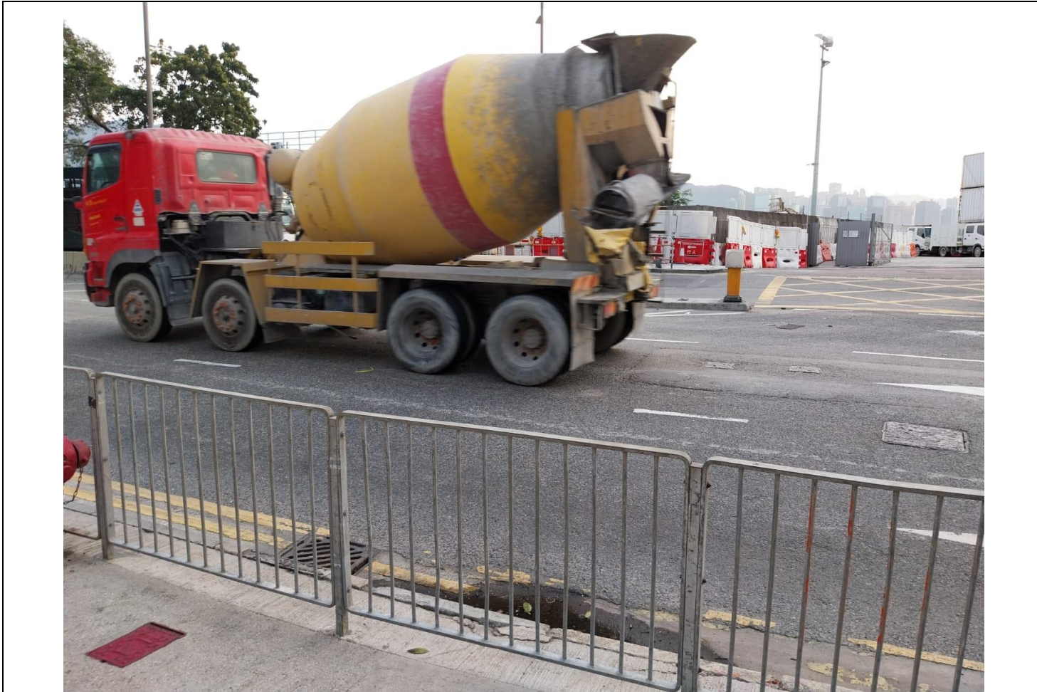
Photo 3 – Road condition along Cha Kwo Ling Road next to station AM4(B) (Taken on 02 Mar 2023)
