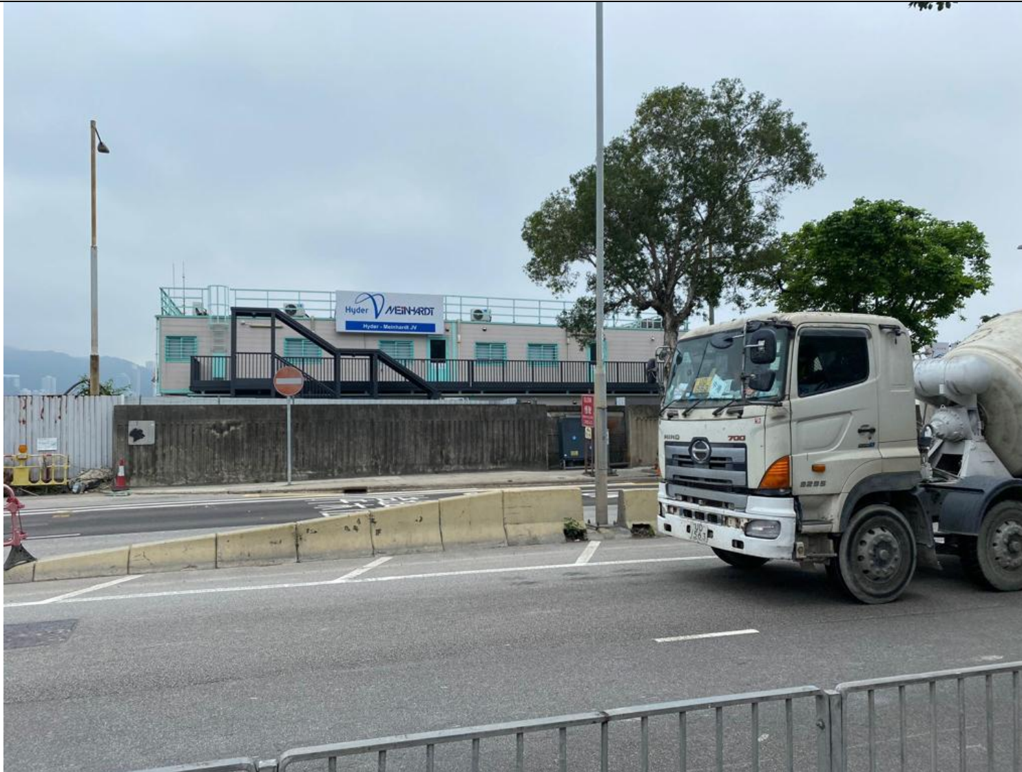
Photo 3 – Road condition along Cha Kwo Ling Road next to station AM4(B) (Taken on 31 May 2023)
