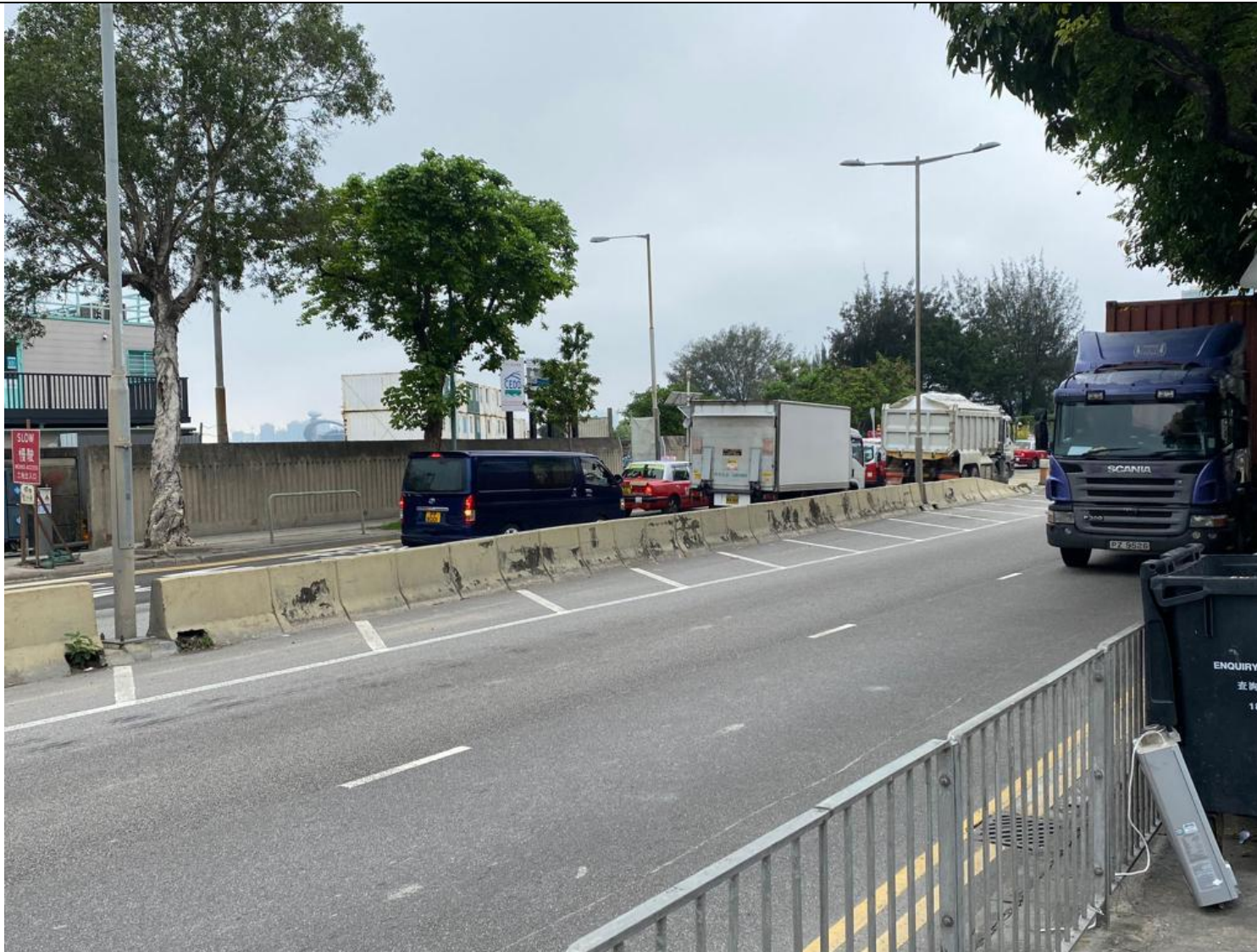
Photo 1 – Road condition along Cha Kwo Ling Road next to station AM4(B) (Taken on 31 May 2023)
