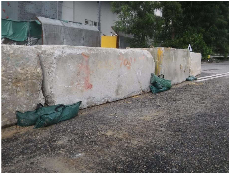
Bunding is provided to prevent the surface runoff.
