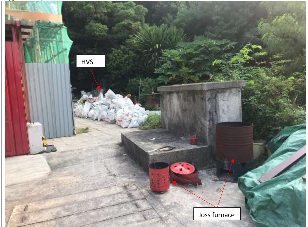
Photo 2 – The HVS was swallowed by bags of dusty materials and the joss furnace located near the HVS. (Taken on 29 Sep 2021)
