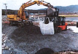
Rubble being added to GEONIA® Ton Bag Anchor
