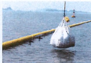
GEONIA® Ton Bag Anchor being installed
