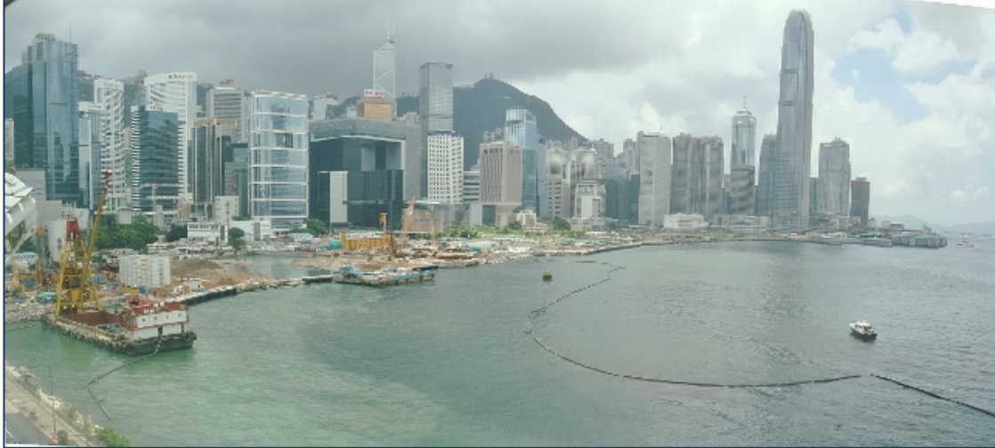
Central – Wan Chai Bypass - seawall separation using heavy non-woven geotextile Bontec SNW120
