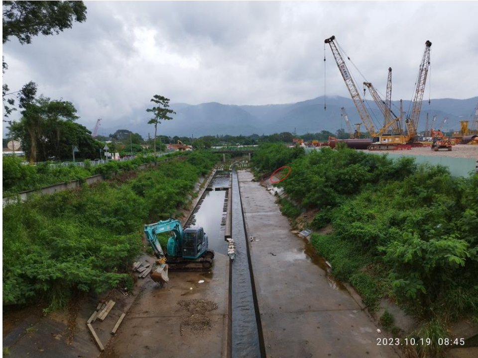
Monitoring Location – P01 (19 th October 2023)
