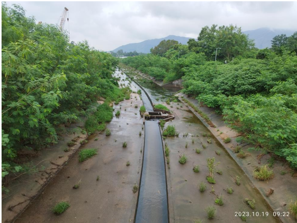
Monitoring Location – P08 (19 th October2023)
