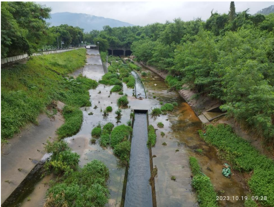
Monitoring Location – P12 (19 th October2023)
