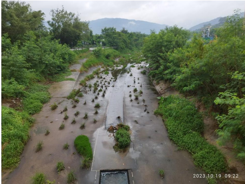
Monitoring Location – P09 (19 th October2023)
