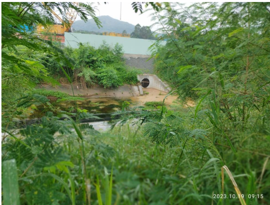
Monitoring Location – P06 (19 th October2023)
