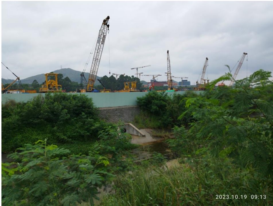
Monitoring Location – P05 (19 th October2023)
