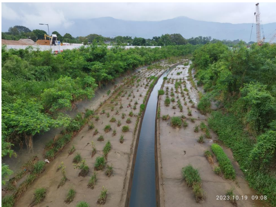
Monitoring Location – P03 (19 th October2023)
