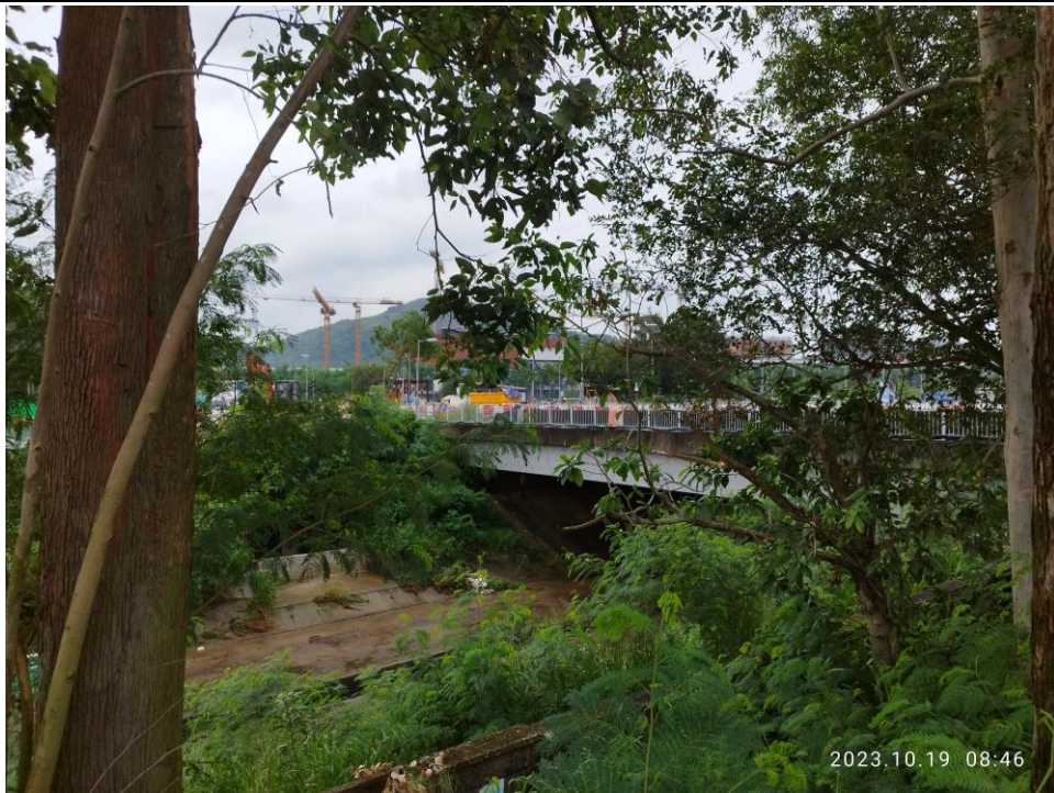
Monitoring Location – P02 (19 th October 2023)
