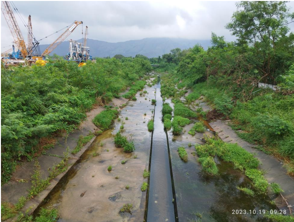
Monitoring Location – P11 (19 th October2023)
