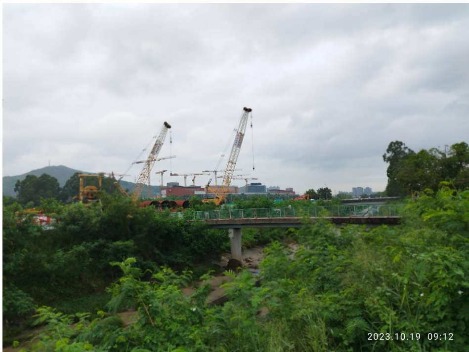
Monitoring Location – P04 (19 th October2023)
