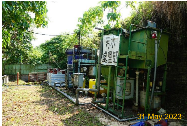
Photo 2 Wastewater treatment facilities (AquaSed, sedimentation tanks) inside the site (near discharge outlet to the northern ditches)
