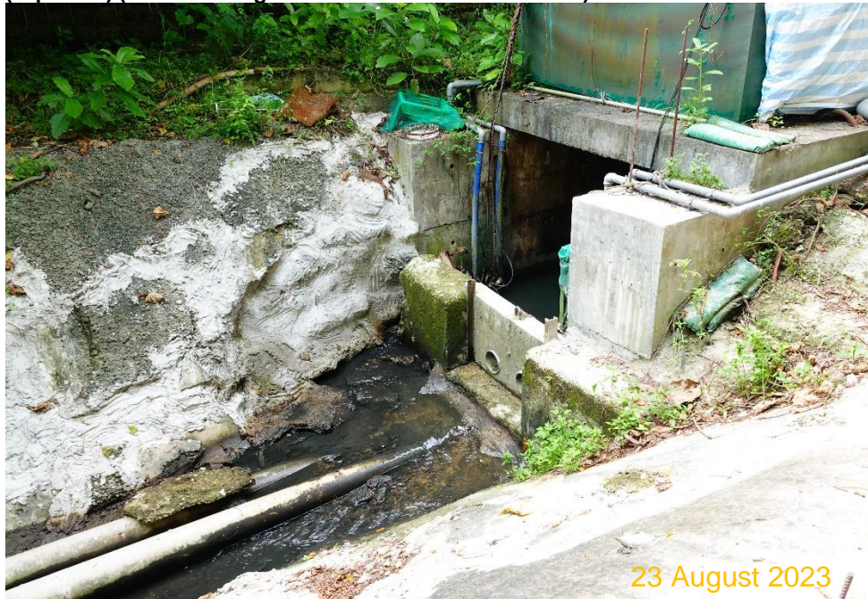
Photo 2 Wastewater treatment facilities (AquaSed, sedimentation tanks) inside the site (near discharge outlet to the northern ditches)
