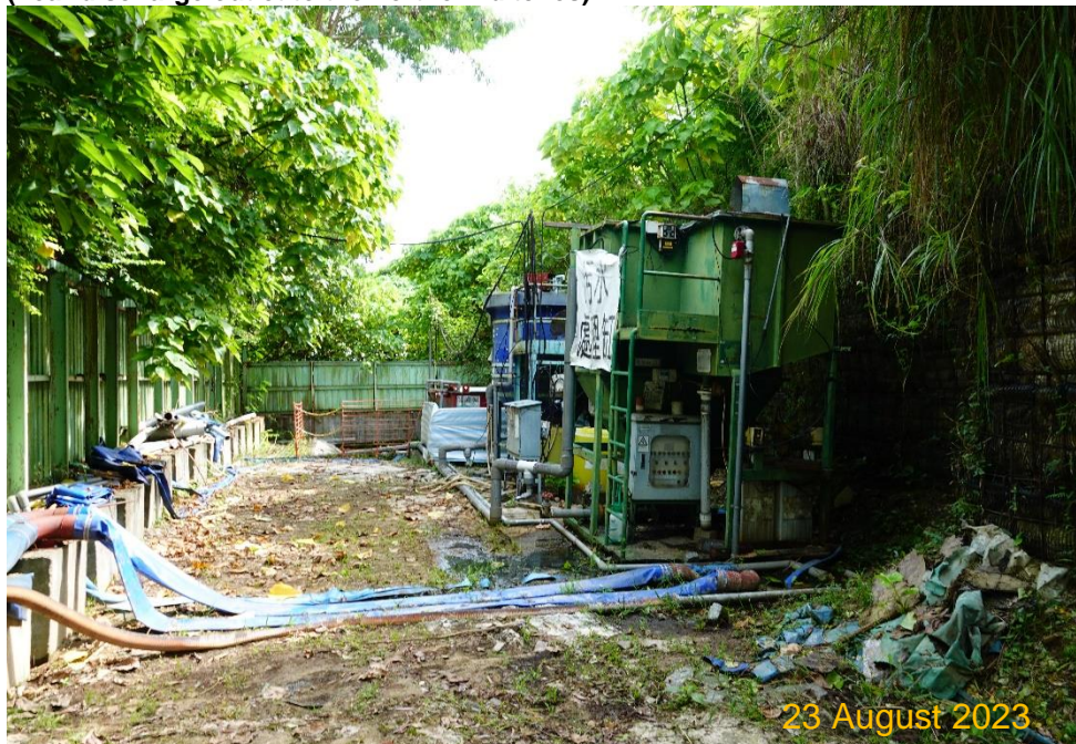
Photo 2 Wastewater treatment facilities (AquaSed, sedimentation tanks) inside the site (near discharge outlet to the northern ditches)
