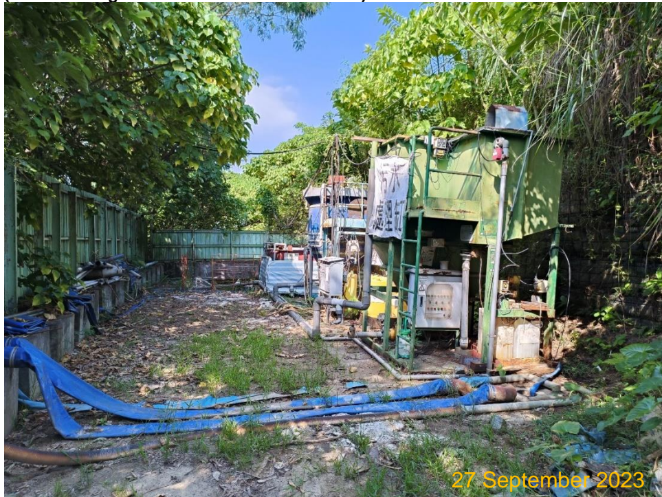
Photo 2 Wastewater treatment facilities (AquaSed, sedimentation tanks) inside the site (near discharge outlet to the northern ditches)
