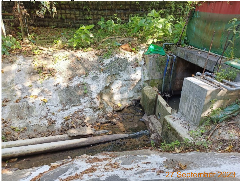
Photo 2 Wastewater treatment facilities (AquaSed, sedimentation tanks) inside the site (near discharge outlet to the northern ditches)
