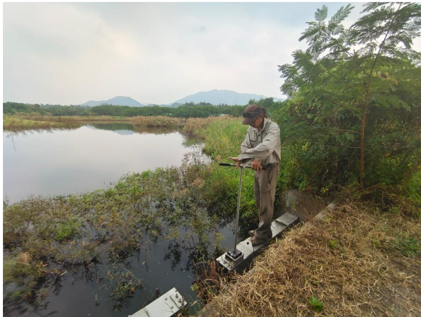
Photo 5 Water level control and mixing water between Cells
