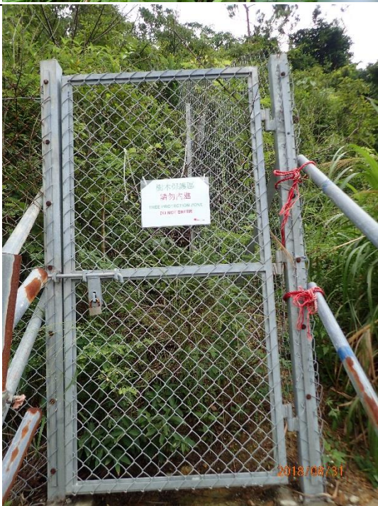
Photo 3 – Current situation of fencing and warning sign
