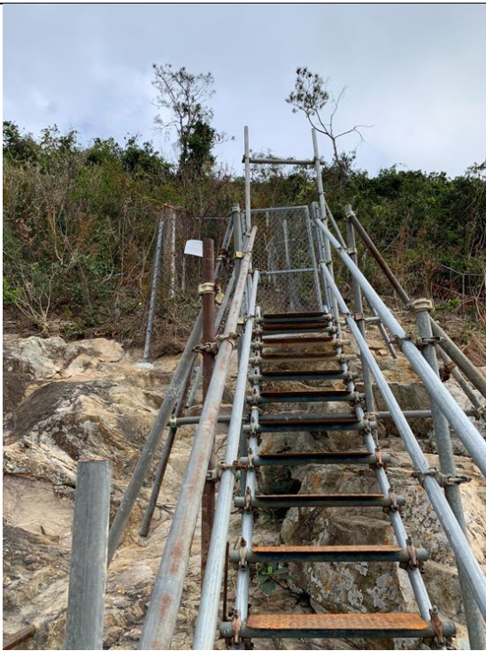
Photo 2 – Current situation of fencing and warning sign
