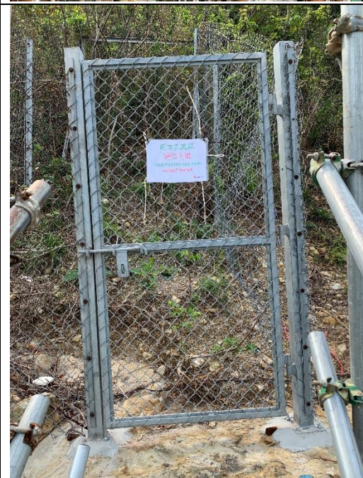
Photo 2 – Current situation of fencing and warning sign
