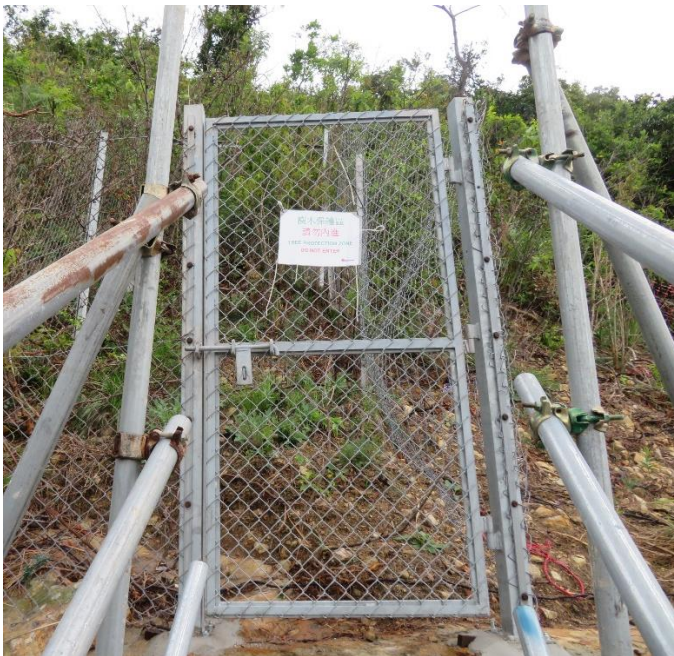
Photo 2 – Current situation of fencing and warning sign
