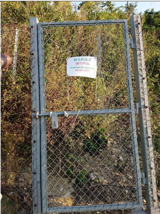
Photo 2 – Current situation of fencing and warning sign
