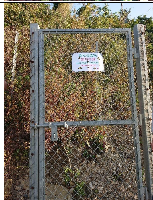
Photo 2 – Current situation of fencing and warning sign
