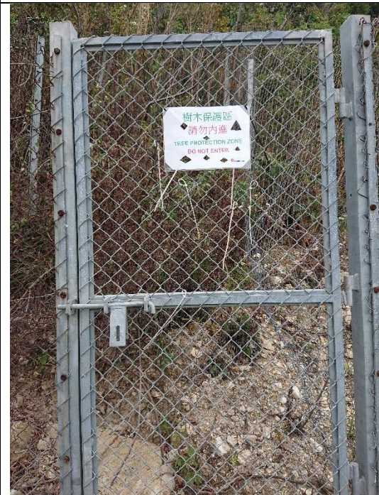
Photo 2 – Current situation of fencing and warning sign
