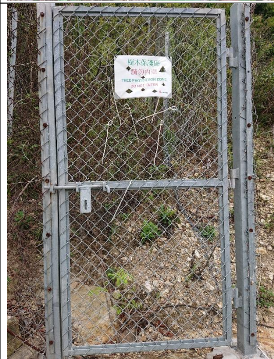
Photo 2 – Current situation of fencing and warning sign
